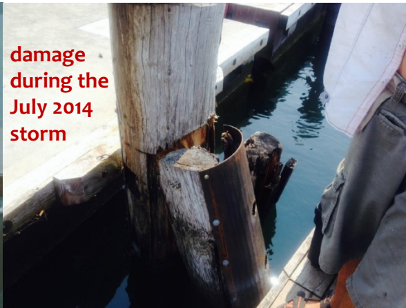
Breakwater damages at a marina on Okanagan Lake (Source: ????? Marina Expansion and Breakwater Repairs - Environmental Assessment, Ecoscope Environmental Consultants Ltd., 2016)
