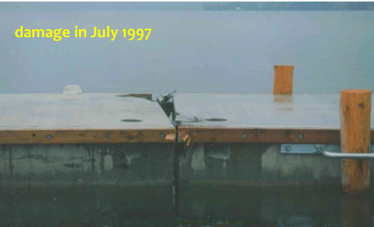
Breakwater damages at a marina on Okanagan Lake (Source: ????? Marina Expansion and Breakwater Repairs - Environmental Assessment, Ecoscope Environmental Consultants Ltd., 2016)
