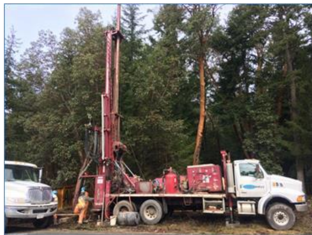
Drilling new observation well on Empress Road, Cobble Hill, B.C. Photo credit: Graeme Henderson
