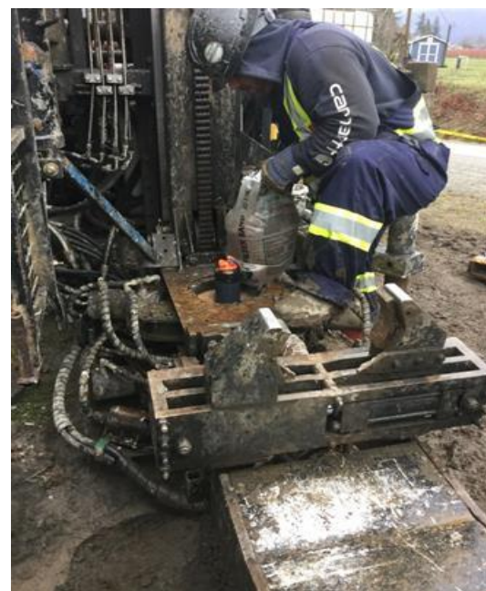
OW465, showing well construction.
