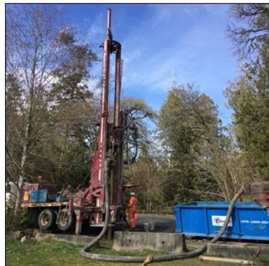
Drilling observation well on Deloume Road, Mill Bay, B.C. Photo credit: Graeme Henderson
