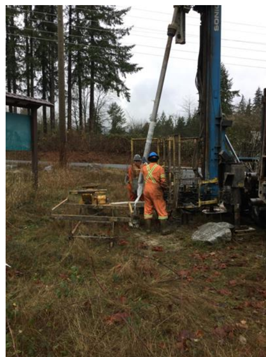
Drilling OW463 with sonic drilling method. Photo credit: Bryan Jackson
