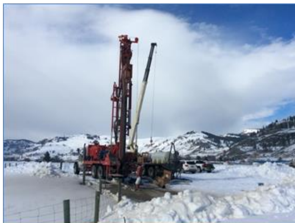
Drilling new observation well, Midway, B.C. Photo credit: John Pogson
