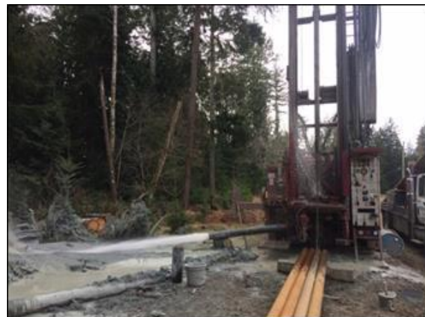
Drilling observation well on Phillips Road, Sooke, B.C.
