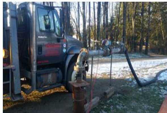
Conducting a pumping test at Steele Park.
