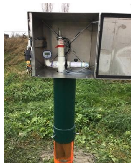
OW461 showing wellhead modification. Photo credit: Michele Lepitre
