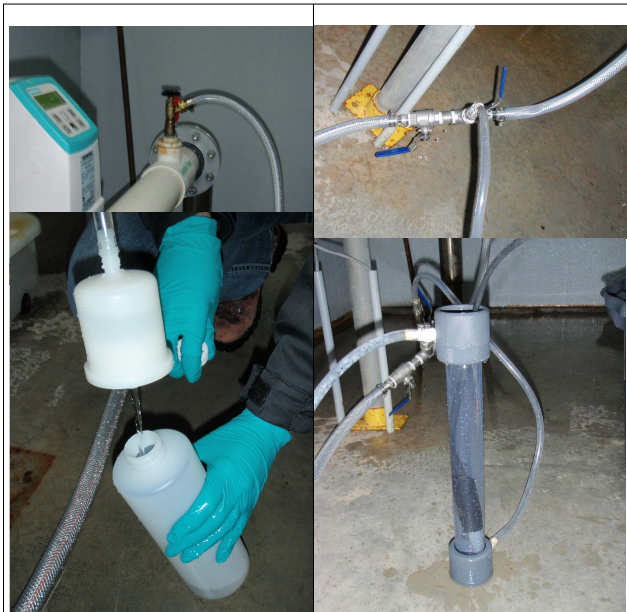
Figure 12: Example sampling set-up. Clockwise from top left: Sample point; discharge line; flow cell; sampling with in-line filter.
