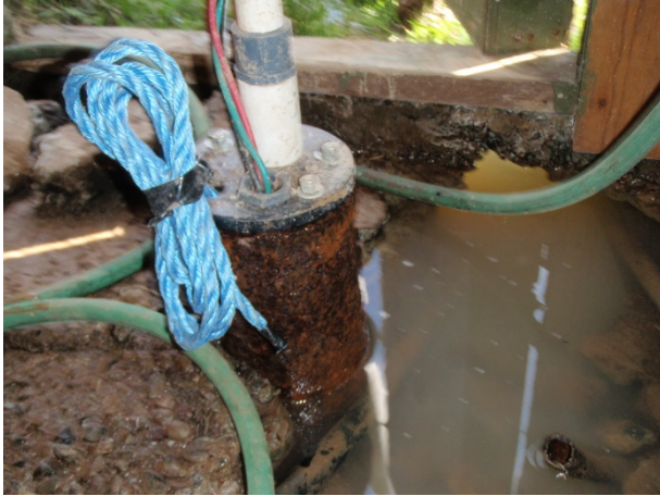
Figure 28: Excavation of materials around the casing allowed standing water to accumulate around this well head. Rodents also inhabited the pump house which was in poor repair. Groundwater samples from the well indicated concentrations of total coliform 880 CFU/100 mL and E. coli 3 CFU/100 mL.
