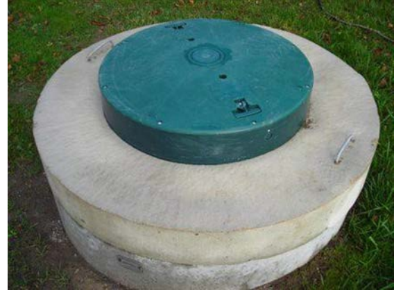
Figure 33: A proper cap/cover should be water-tight and prevent entry of water and foreign matter. Dug wells capture shallow groundwater and are naturally more vulnerable to contamination. The groundwater typically requires some form of disinfection, such as ultraviolet (UV), to remove potentially harmful bacteria and pathogens (Photo source: Regional District of Nanaimo, WellSmart, 2018).
