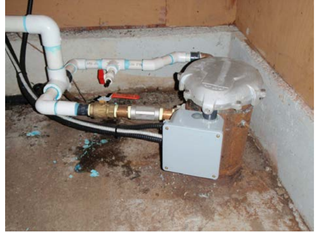
Figure 29: Ensuring the well head has 30 cm or more stickup above the floor of the pump house and keeping the pump house clean, free of potential contaminants, and maintained to prevent entry of vermin including rodents and insects helps ensure the groundwater remains safe to drink.
