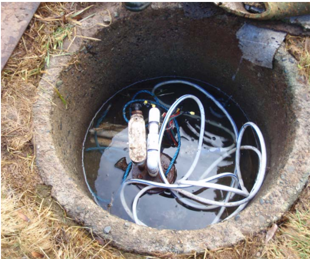
Figure 30: Below ground enclosures must have a water-tight lid and interior drain to prevent accumulation of standing water around the well. Groundwater from this drilled well contained total coliform 20 CFU/100 mL indicating it had been contaminated by entry of surface water.
