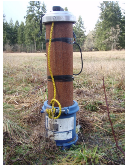
Figure 31: A registered qualified well driller or well pump installer can be hired remove a well pit or enclosure. In this case, a water-tight coupling was attached to the casing to raise the casing stickup above ground and prevent unintended entry of contaminants into the well.
