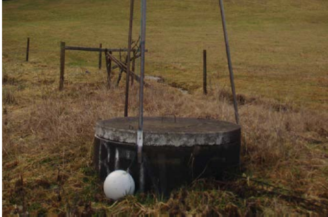
Figure 32: The design of the access port on the top of this excavated (dug) well allows rain and contaminants to enter the well. The site is also located in a cattle pasture with no setback of animals from the well. The groundwater sample had total coliform 87 CFU/100mL and E. coli 5 CFU/100 mL.
