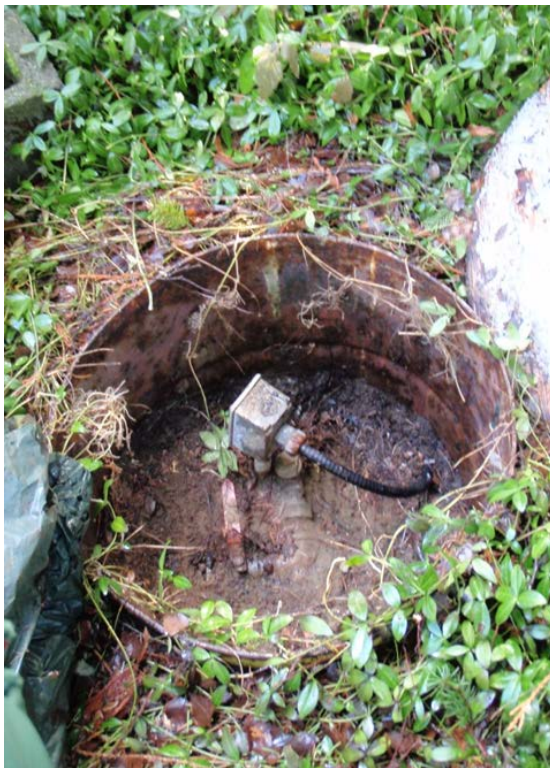
Figure 34: This sanitary seal well cap was covered in saturated soil in an outside enclosure. The groundwater sample had total coliform 34 CFU/100mL and E. coli 19 CFU/100 mL.
