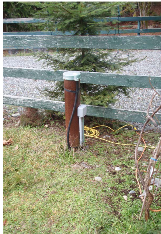
Figure 35: Ensuring the well is properly capped and not buried below ground protects the well from potential contaminants. Probable sources of contamination such as septic systems, animal paddocks, coops and manure storage areas should be set back a minimum of 30 m from the well.
