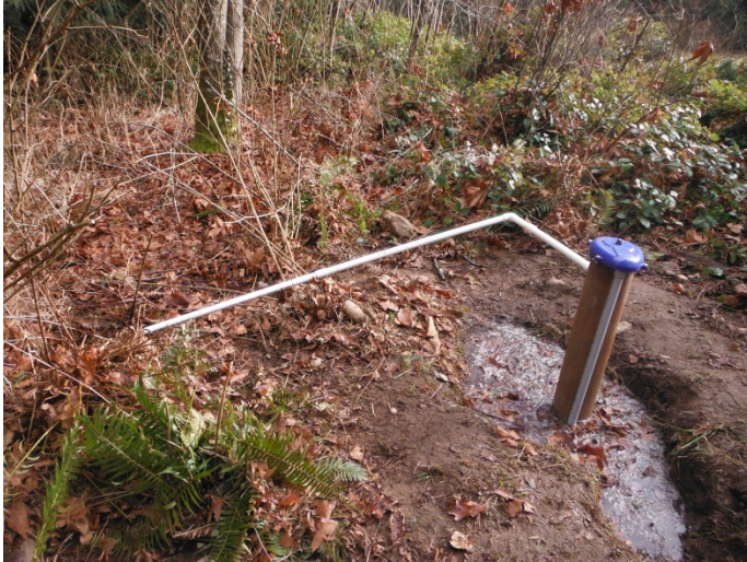
Figure 36: Drain line and ditching installed to direct water away from this flowing artesian well put it at risk from erosion of materials around the casing, and loss of pressure in the aquifer. Under the Water Sustainability Act, Section 53 artesian flow must be controlled, there must be the ability to stop the flow indefinitely, and the overflow pipe requires a backflow preventer to stop contaminants from re-entering the well.
