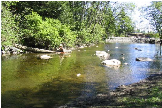
Photo 5. Little Qualicum River boulder-riffle at site D0+370 looking D/S. Note avulsion effects.
