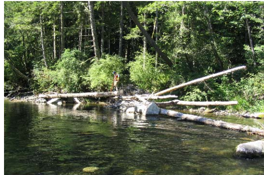
Photo 6. Little Qualicum River LWD failed structure at site C0+757 looking U/S.
