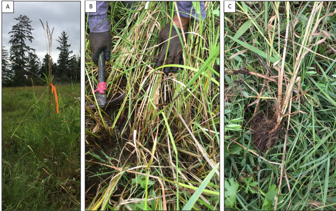
Figure 10- Manual excavation of small patches of reed canary grass. A) Small patches were identified and flagged. B) Crew members from Sellentin's Habitat Restoration and Invasive Species Consulting Ltd. removed small patches using shovels and mattocks. C) Attempts were made to remove the full roots mass and avoid breaking off rhizomes.
