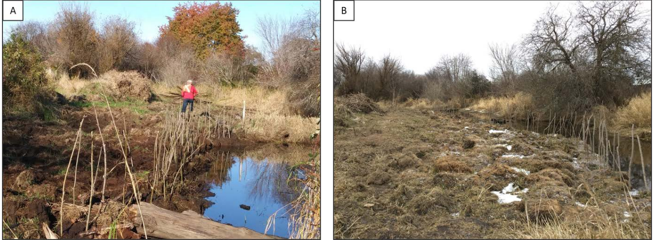
Figure 12- A) Volunteer planting live willow stakes in areas along Mallard Creek where machine excavation had previously occurred. B) Row of live willow stakes along Mallard Creek and area remaining to be planted.
