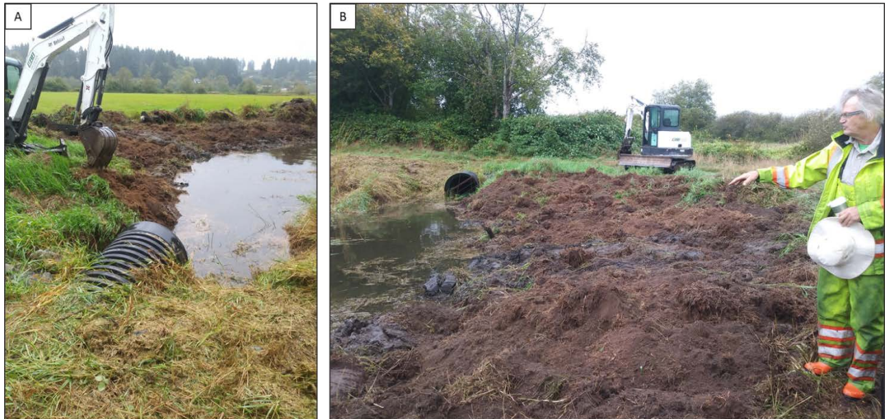
Figure 11- A) Small excavator peeling back mats of reed canary grass (RCG) along Mallard Creek. B) Ernest Sellentin pointing at areas where RCG mats have been peeled back along Mallard Creek
