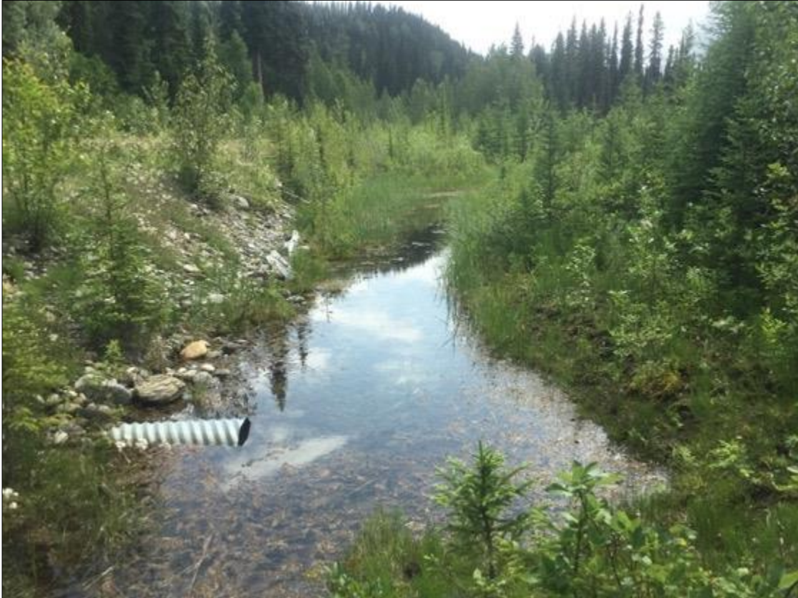
Figure 7. Blocked culvert at site W1
