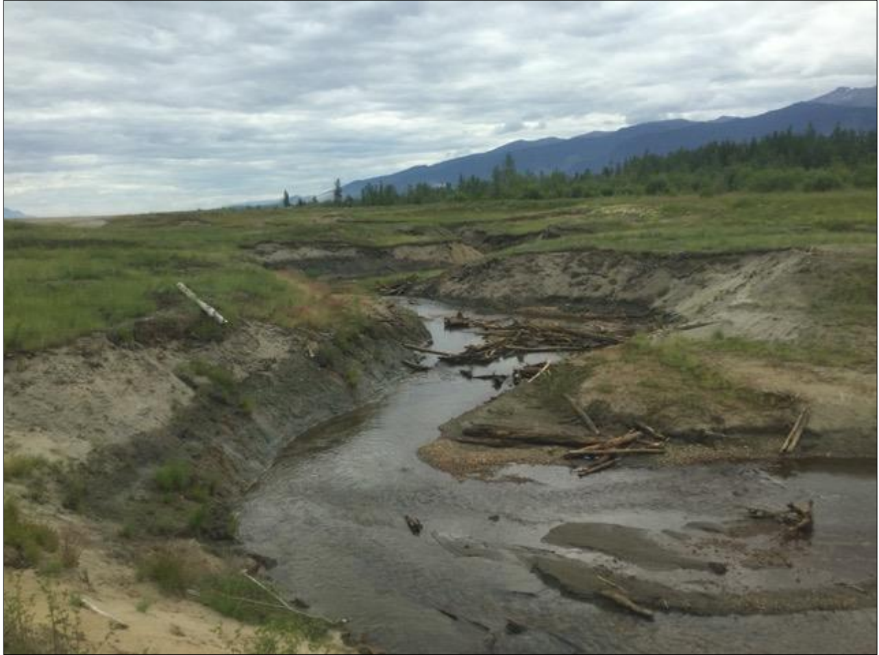
Figure 14. Deep channel created by the headcut at Middle Creek leading to drying of the wetland
