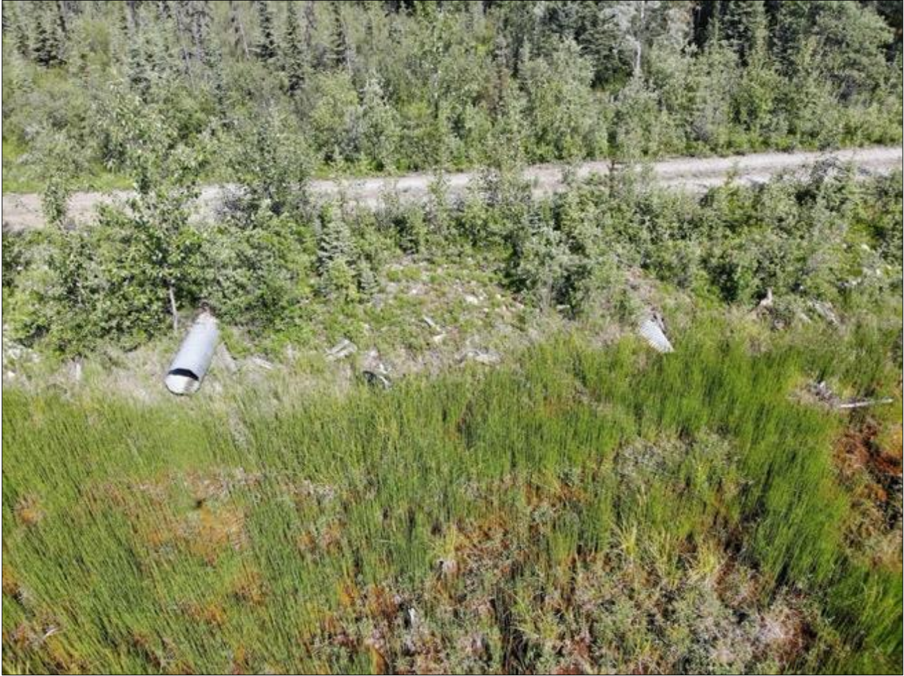
Figure 22. Culverts at site W9. Left culvert is perched high, right culvert is buried
