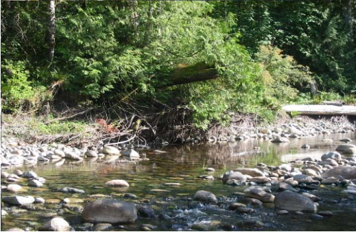
Photo 5. Typical South Englishman pool, note non functional wood and bank scour.
