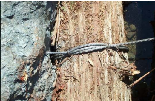
Photo 7. Key ballast secured to log with steel cable using a clove hitch and hog staples.
