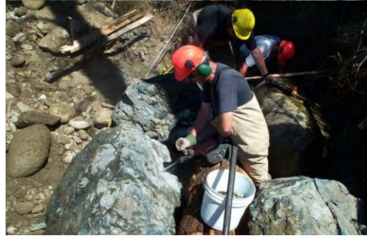
Photo 6. Technician drilling ballast rock with a hammer drill (2003 project).
