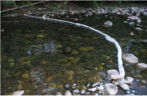
Photo 3. Typical environmental controls (oil boom) installed in the South Englishman River.
