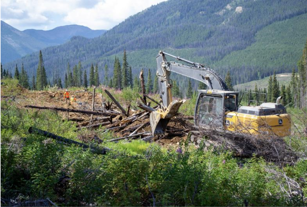
Figure 8.8. The excavator completing some functional restoration by creating a berm of soil and coarse woody debris to break up the sightline along a road segment.
