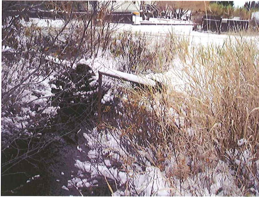
View of inlet. Note the anti-beaver devices.
