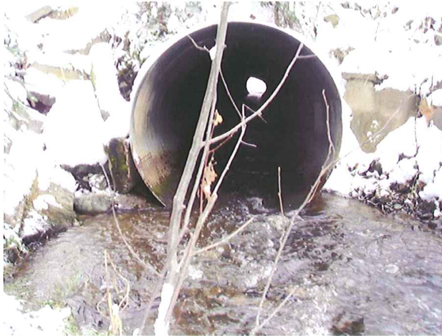
View of inlet.
