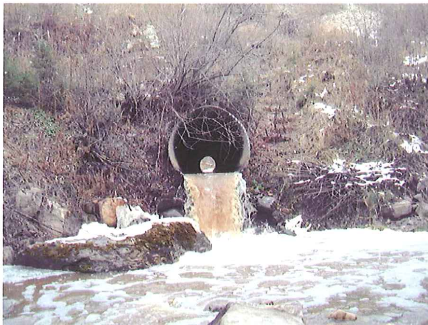
View of outlet.
