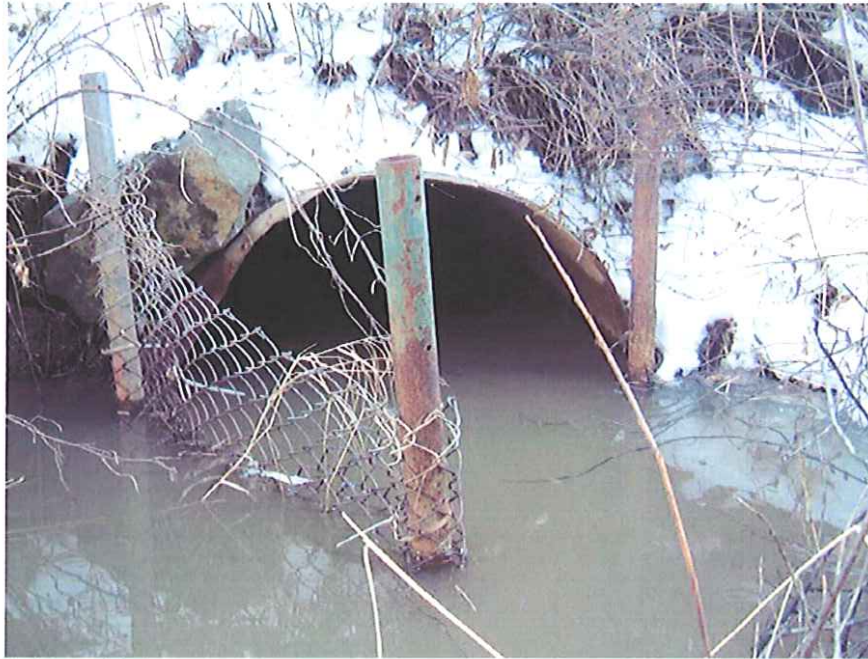
View of inlet.
