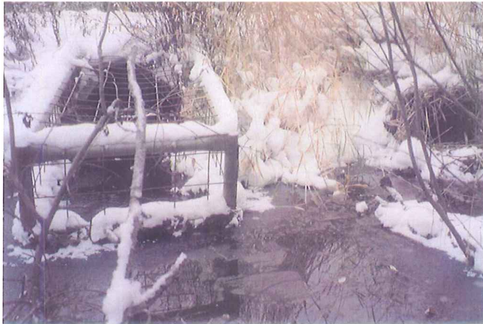
View of inlets.
