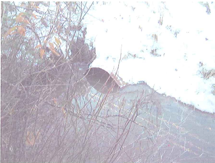
View of outlet.
