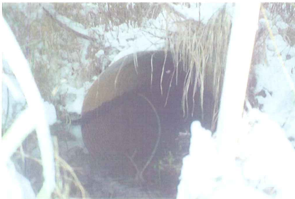
View of outlet.
