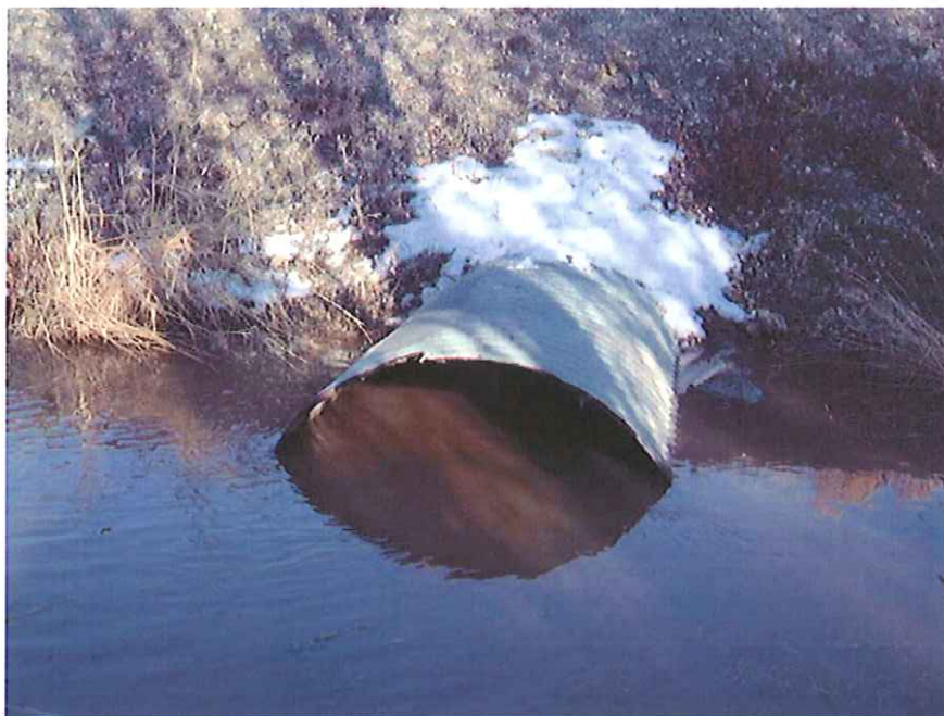
View of right bank inlet.
