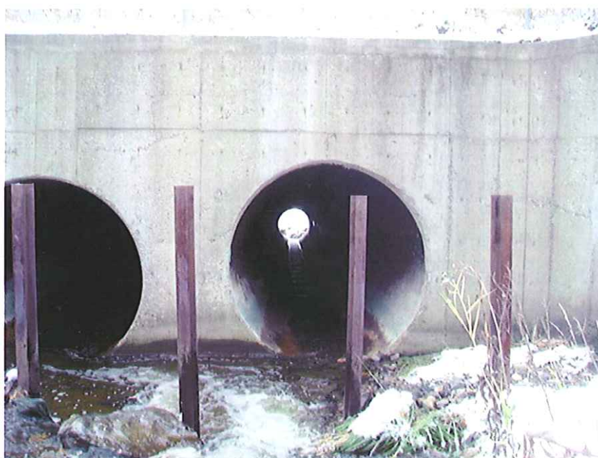
View of right bank inlet.
