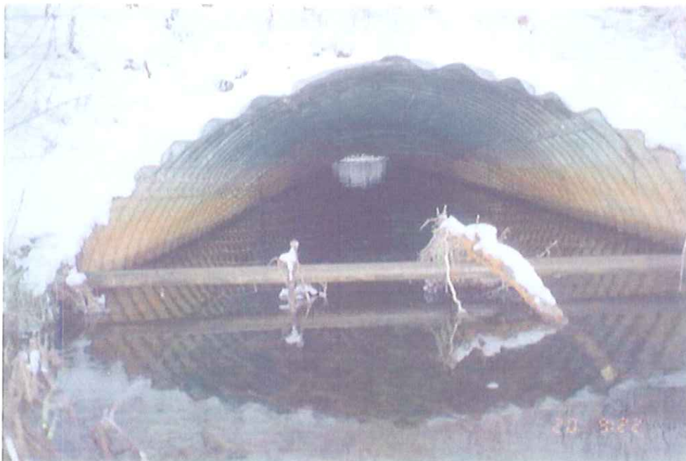
View of outlet.
