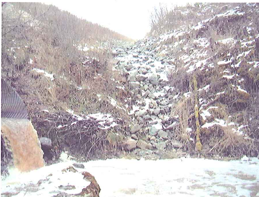
View of outlet and right bank slope.
