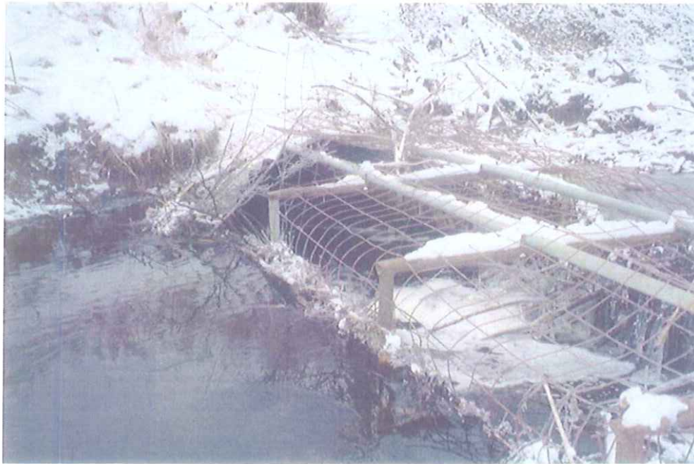
View of inlet.
