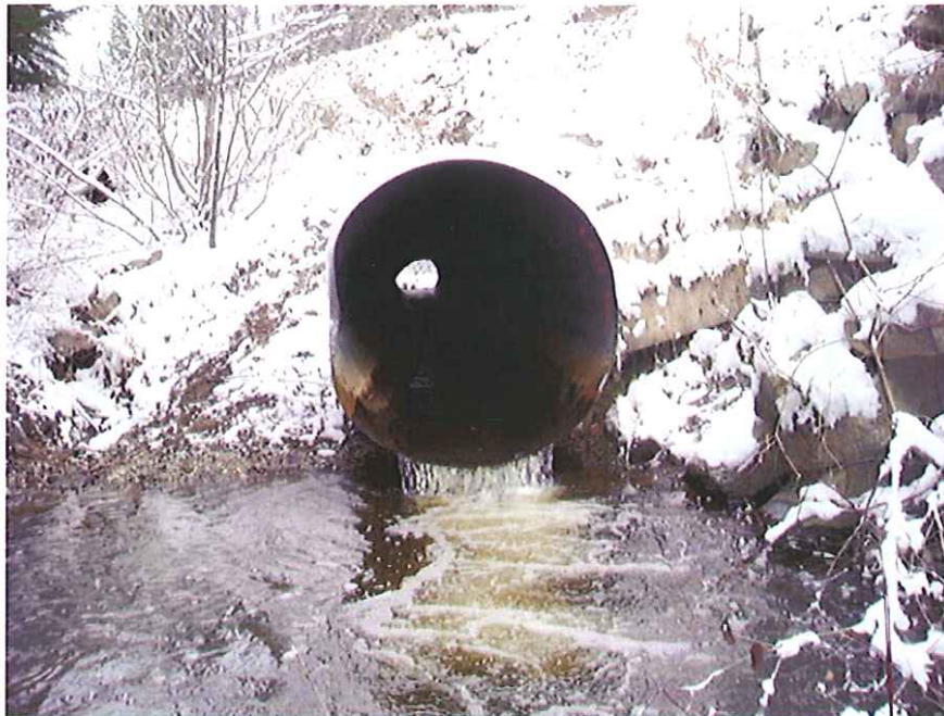
View of outlet.
