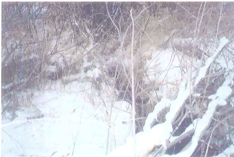
View downstream of outlet.
