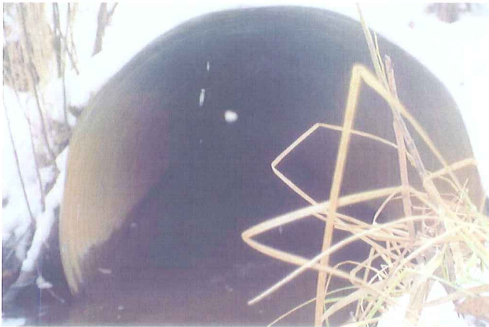
View of inlet.
