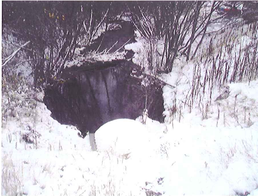
View upstream of inlet.
