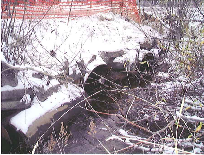
View of middle outlet and right bank outlet.
