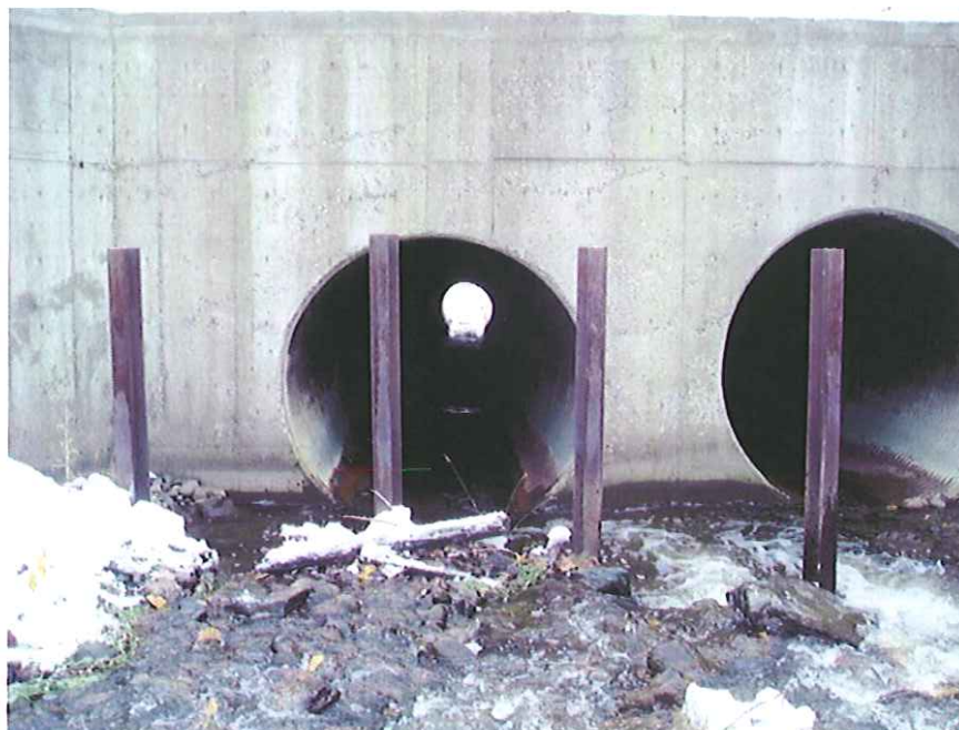
View of left bank inlet.
