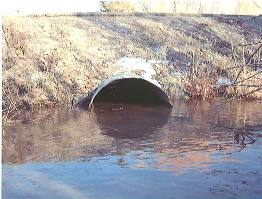
View of left bank inlet.
