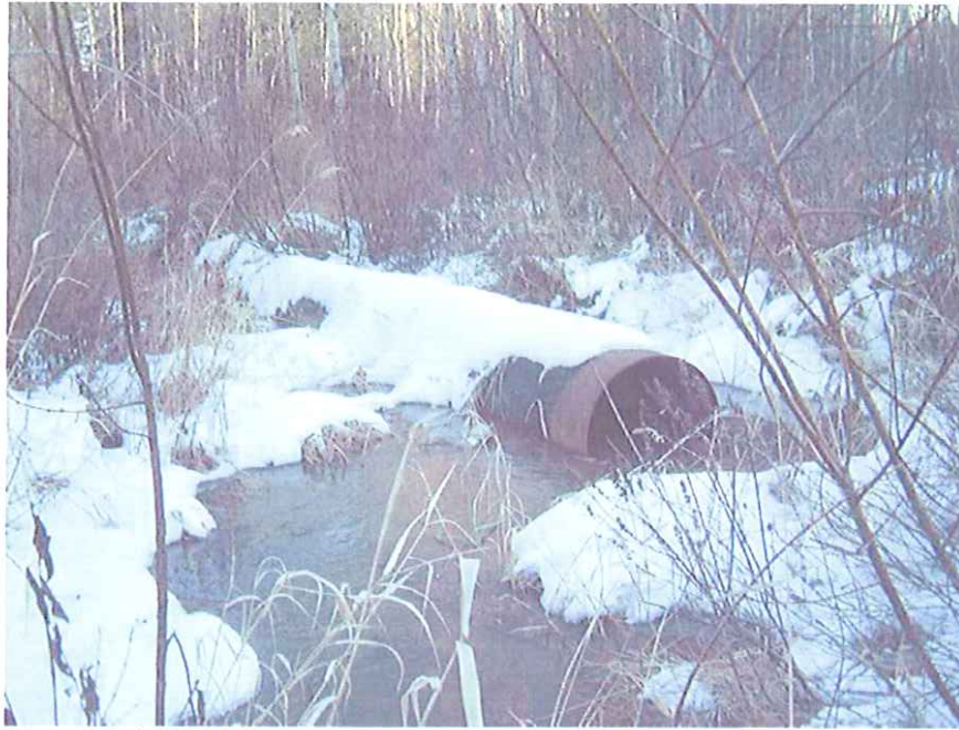
View of old corrugated metal pipe within stream channel.
