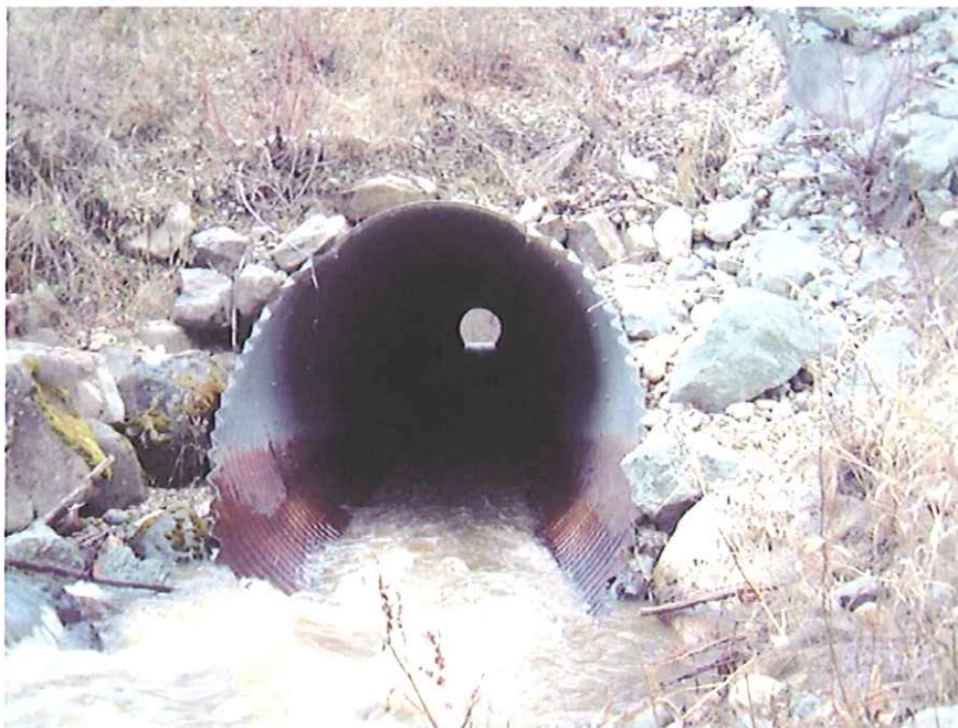
View of inlet.
