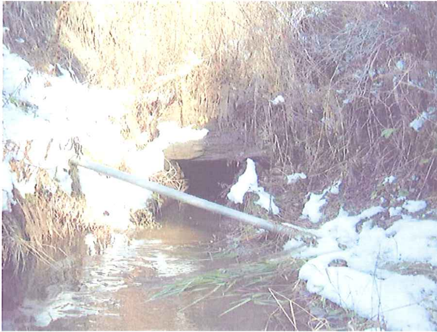
View of inlet
