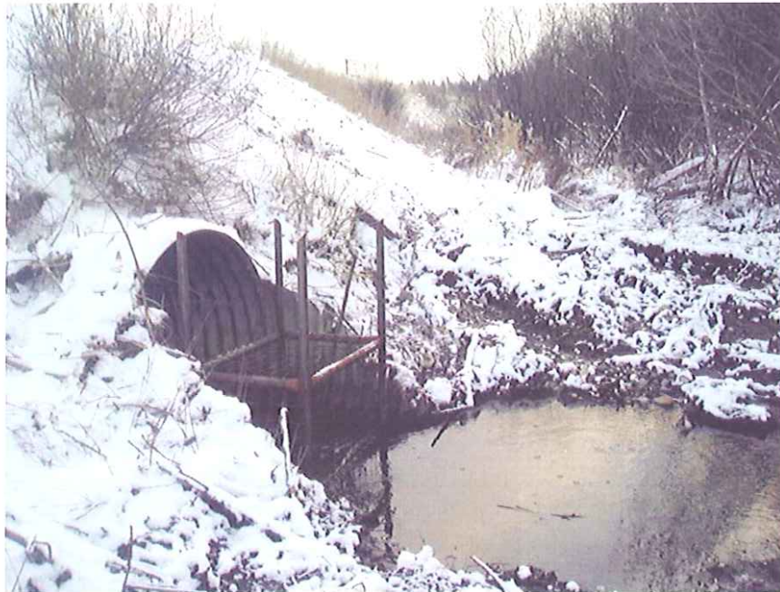
View of inlet
