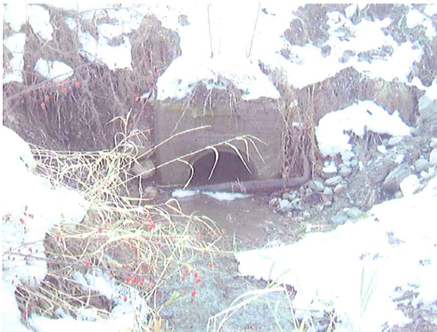
View of outlet.
