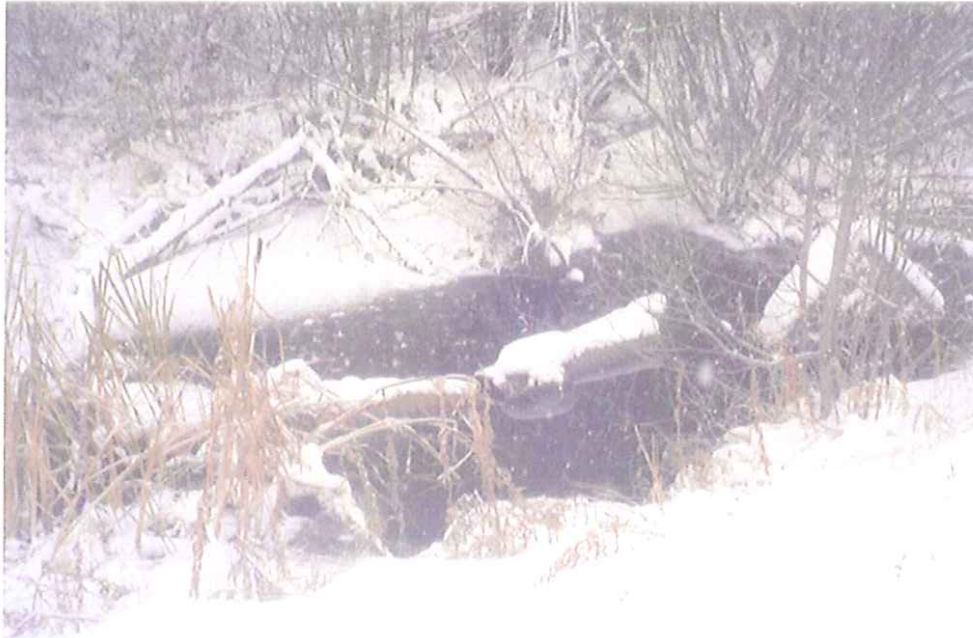
View of old culvert within the stream channel upstream of inlet.
