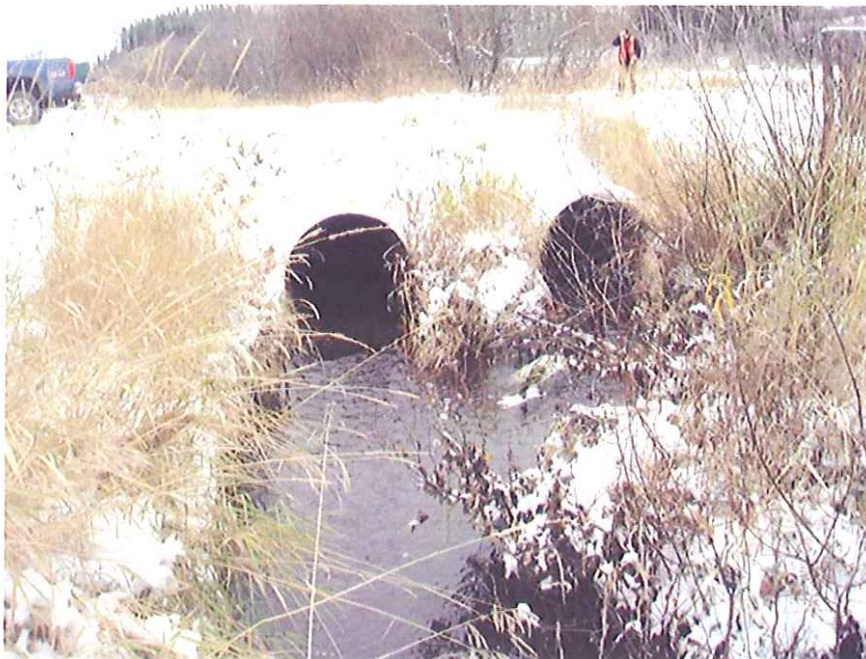
View of outlet.
