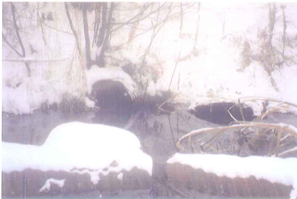
View of old culvert within the stream channel facing inlet.
