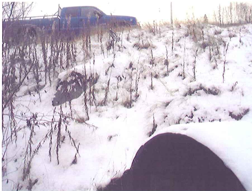
View of outlet
