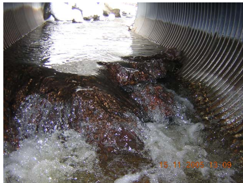
Photo 4 – View looking upstream at riffle in culvert created by large angular boulder from rock-armoured inlet entering culvert.
