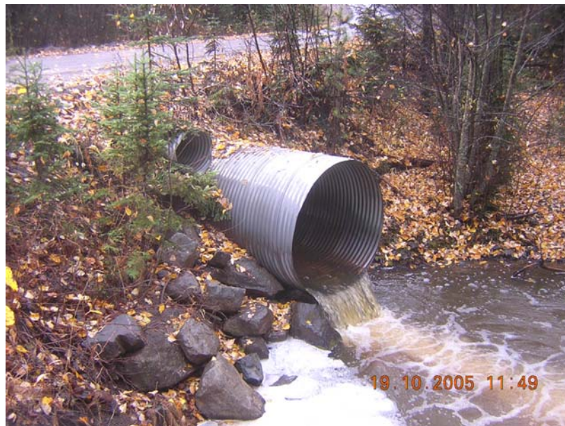
Photo 7 – View of perched culvert outlet and overflow culvert.
