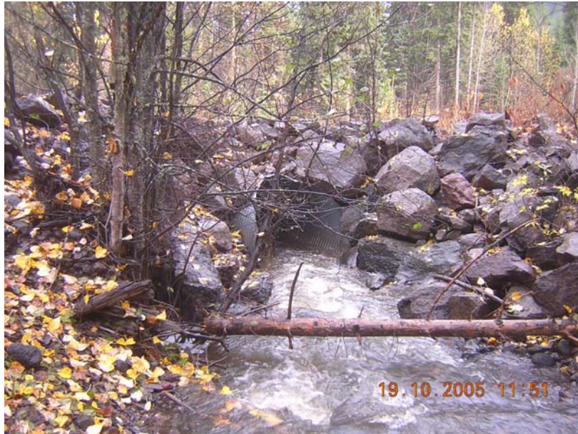
Photo 5 – View looking downstream at rock-armoured culvert inlet.
