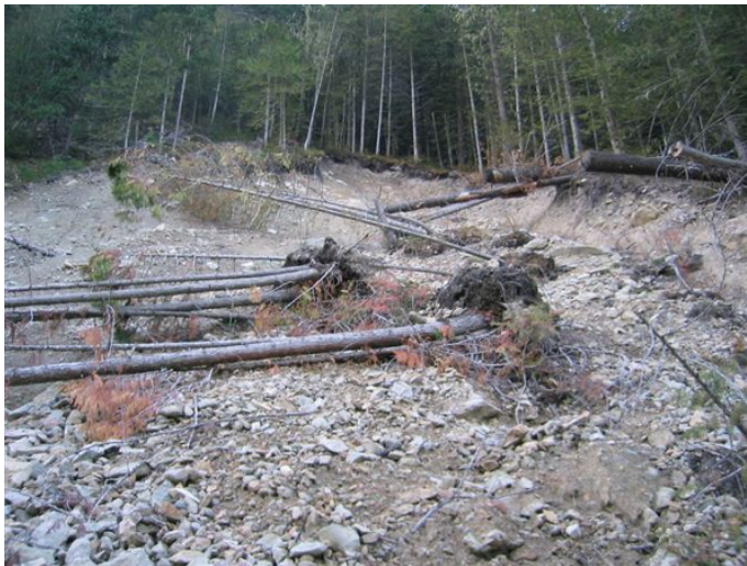
Photo 13. Initiation zone of debris slide that initiated in deep surficial material.
