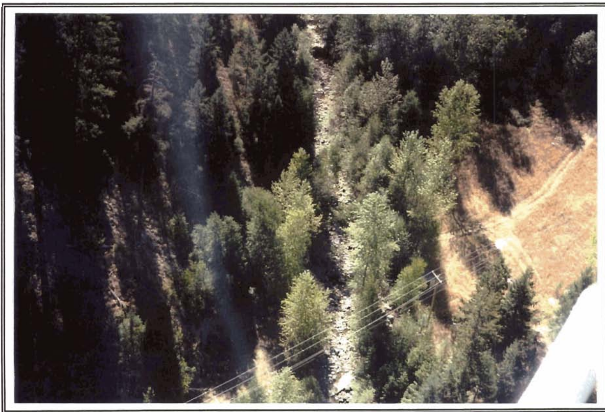
PHOTO KA-2. Reach KA - Overview (RA4, P15)
