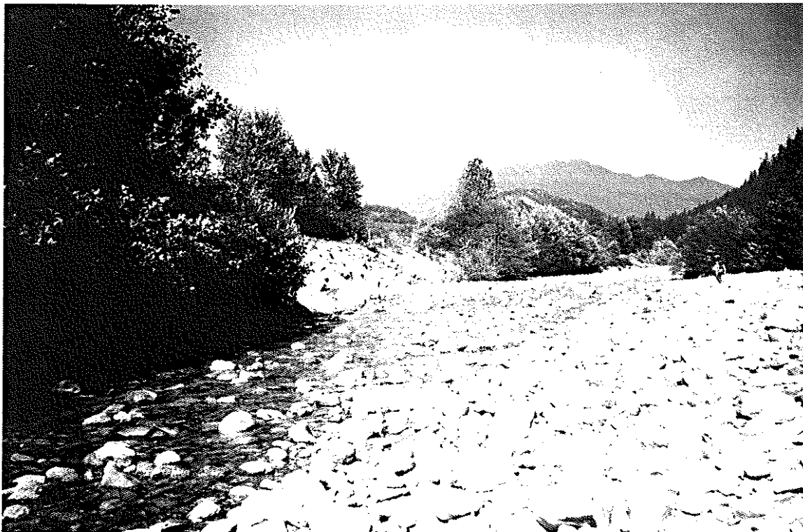
Photograph 10: Upstream view of dike on right bank, channel is trained and has an elongated riffle zone. Potential for restoration to vegetate the banks (Reach 6 - 08/98).
