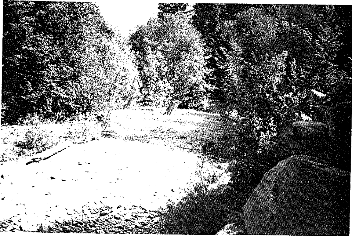
Photograph 10: Upstream view of dike on right bank, channel is trained and has an elongated riffle zone. Potential for restoration to vegetate the banks (Reach 6 - 08/98).
