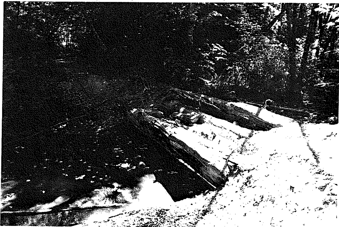
Photograph 19: Foot bridge resulting in sediment deposition to stagnant water upstream (Little Stawamus - 09/98).
