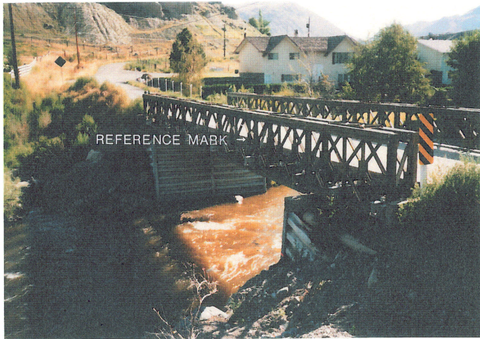
H.W.M. #1 Bonaparte River Bridge at Ashcroft, upstream side.
