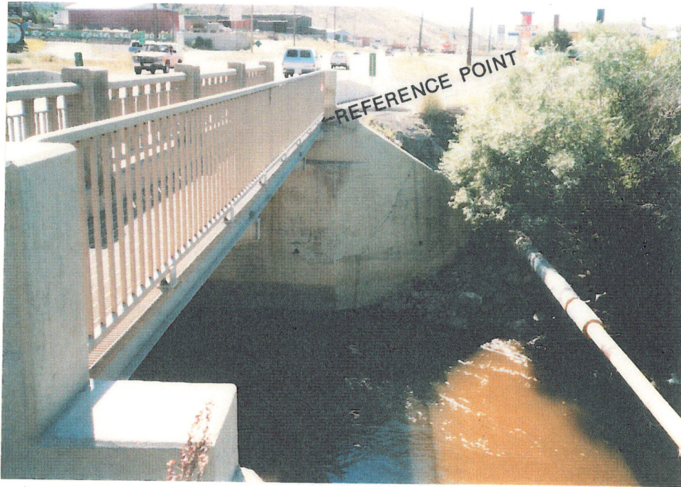
H.W.M. #4 Hwy.#97 Bridge at north end of Cache Creek.
