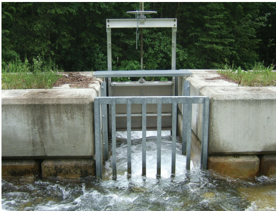
Figure 1. Mutton Creek diversion
