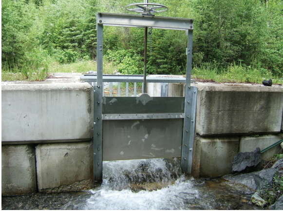
Figure 4. Mutton diversion gate system
