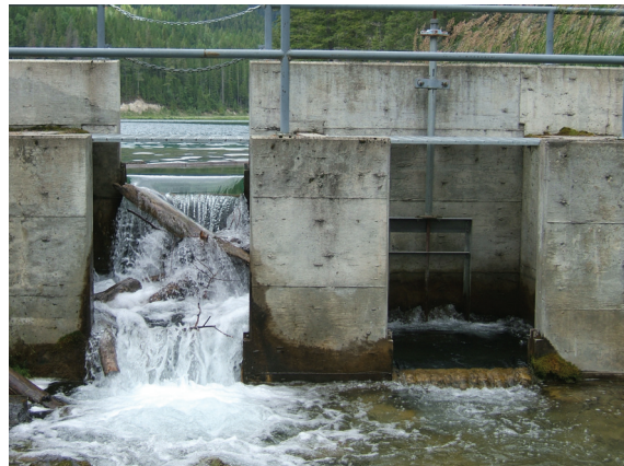
Figure 2. Alces Lake deep water outlet
