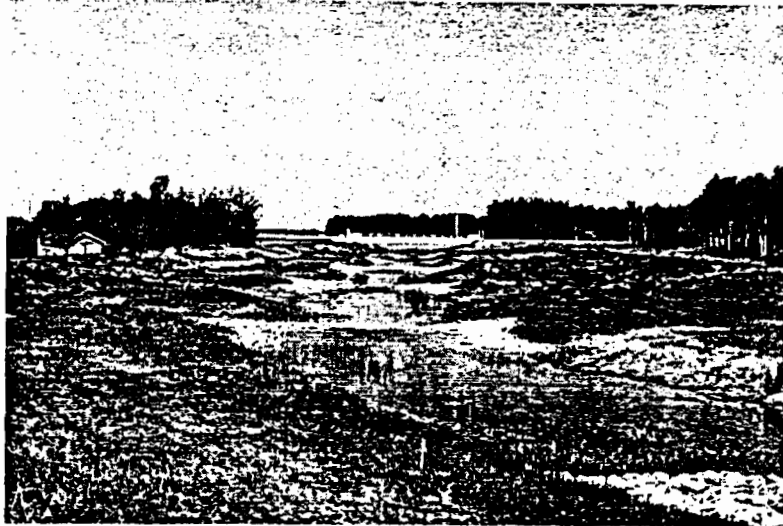
Figure 17: Mink Creek Walleye Spawning Restoration Project 1988, Central Manitoba. The channelized reach 3 years after rock riffles were added. After several bankfull and greater flood events formed downstream pools, the channel has stabilized. The riffles and upstream pools are utilised by spawning walleye.
