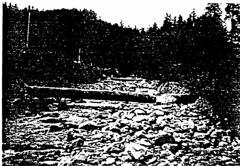
Figure 19: Oulette Creek 1982, Howe Sound, BC. In the first three years following channelization, the single log drop structures added to the uniform channel were undercut. Alternating single boulder drop structures were buried in deep scour holes formed immediately below the structure crests as there was no downstream riffle to convey the flows away from the structure.
