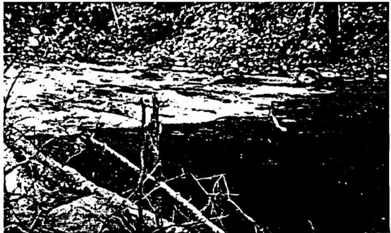
Figure 7: Chapman Creek Restoration Project 1995, Strait of Georgia, BC. Coarse gravel bars have in-filled in the upstream pool that are utilised by spawning salmon. The downstream slope and crest elevation were not changed by greater than bankfull flood flows.
