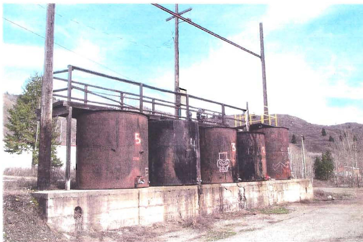
Photograph 8: Large, old, rusted, unidentified ASTs on west side of Granby Road (on inferred former smelter site). Looking east. March 2003
