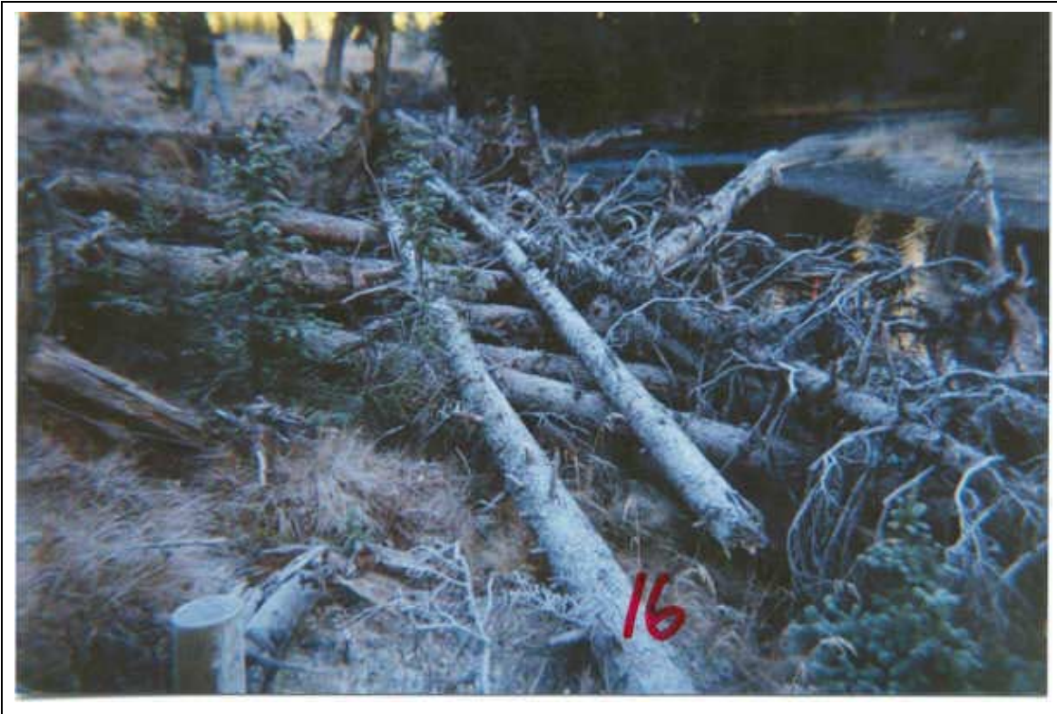
Plate 37 Live stakes planted along bank, Maiyuk Creek (October 23-26, 2000). Note white tops of stakes.
