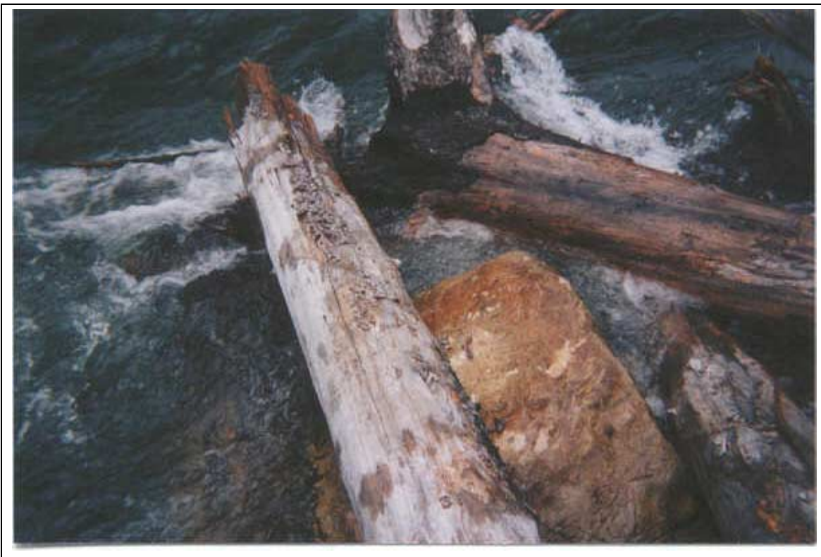
Plate 26 View toward centre of channel showing ballast rock, triangular logjam MF-01, Middle Fork of the White River (July 22, 2000).
