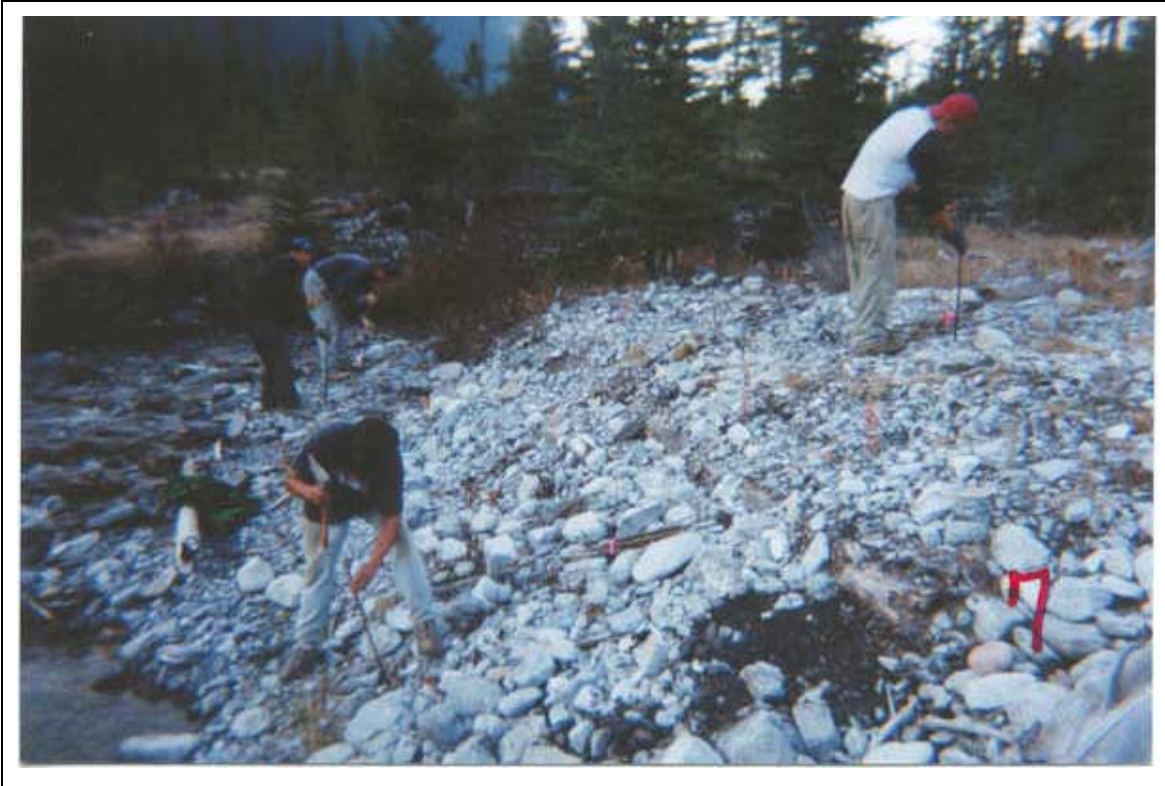
Plate 43 Live stakes planted along bank, Klookuh Creek (October 23-26, 2000). Note white tops of stakes.
