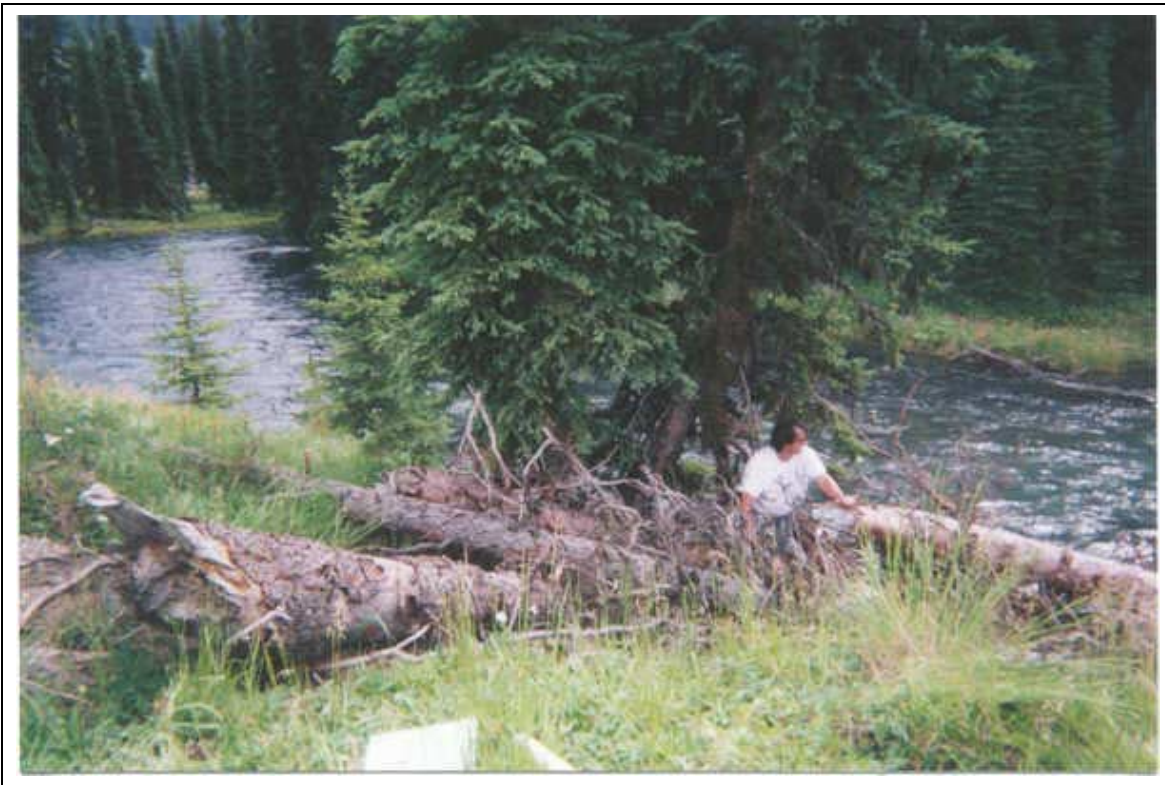
Plate 22 View of channel upstream from structure; site MY-01, Mayuik Creek (July 22, 2000). Jim King as scale.
