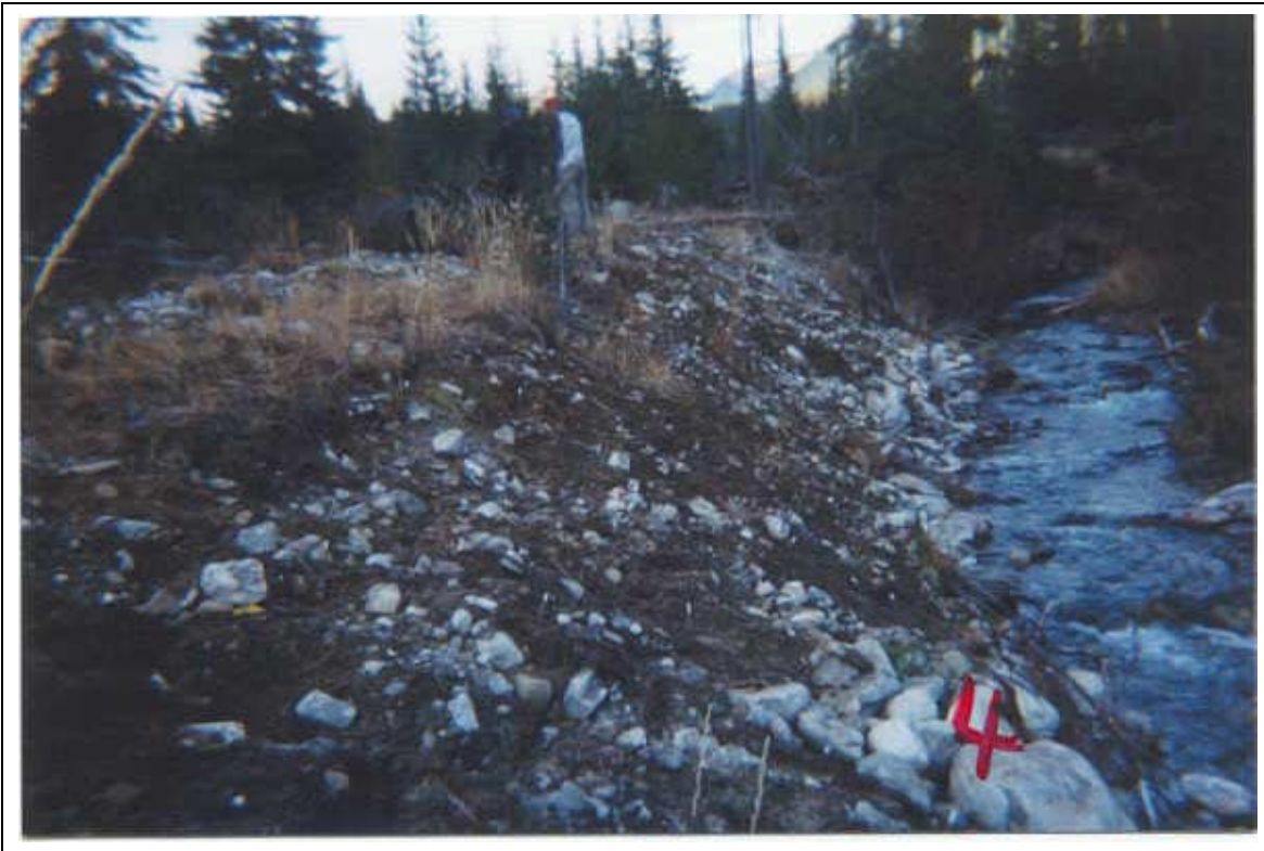
Plate 40 Live stakes planted along bank, Klookuh Creek (October 23-26, 2000). Note white tops of stakes.
