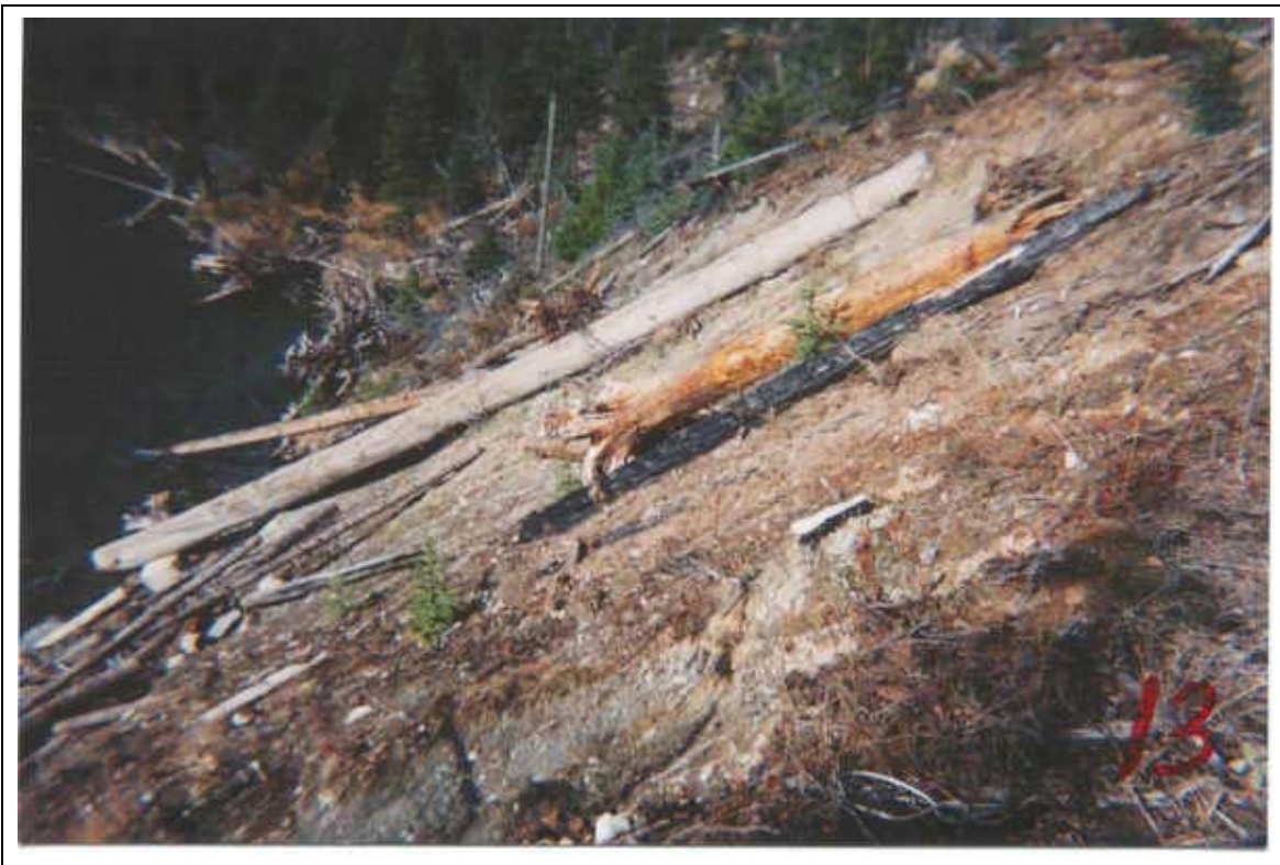
Plate 38 Live stakes planted along bank slope, Middle Fork of the White River (October 23-26, 2000). Note white tops of stakes.
