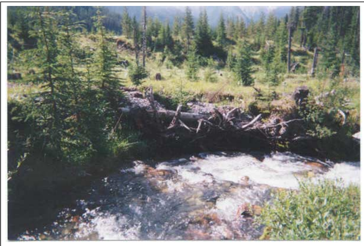
Plate 8 View across and downstream at tree revetment; site KK-04, Klookuh Creek (July 22, 2000).
