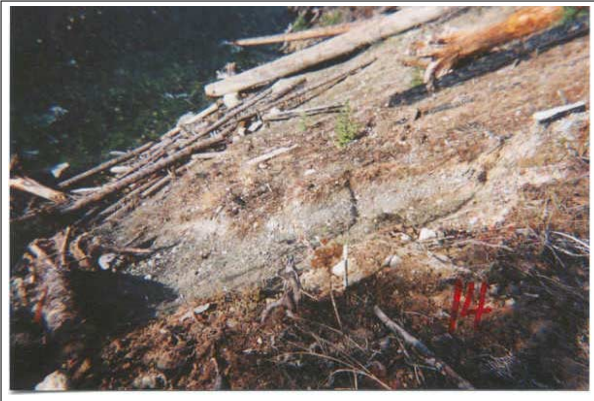
Plate 39 Live stakes planted along bank, Middle Fork of the White River (October 23-26, 2000). Note white tops of stakes.
