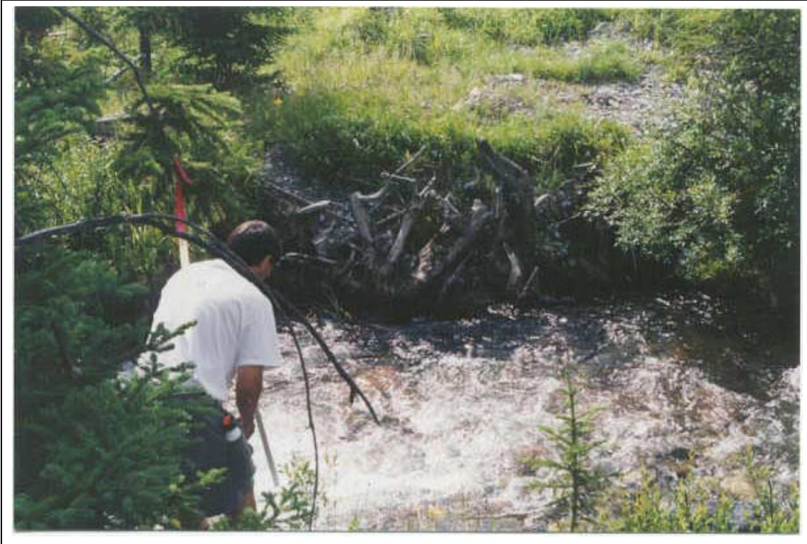
Plate 3 View across stream channel at tree revetment; site KK-02, Klookuh Creek (July 22, 2000). Jim King as scale
