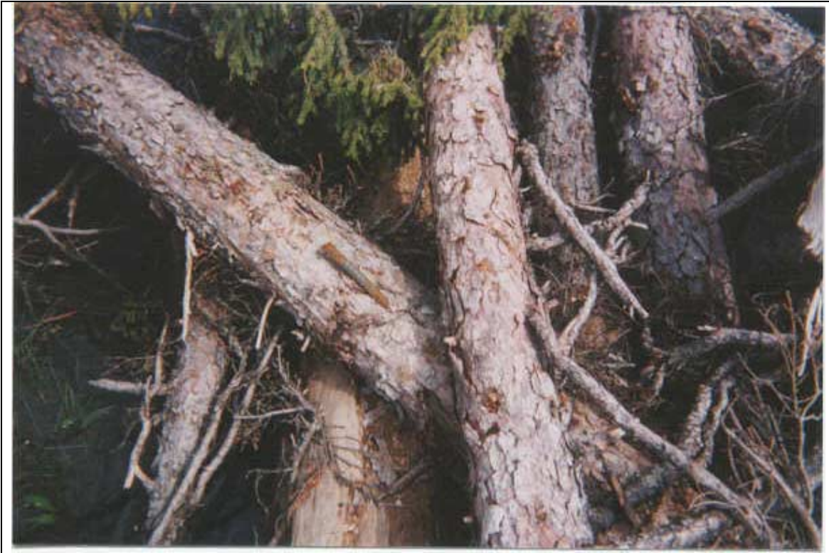
Plate 21 View of typical rebar pin used to secure spruce logs, site MY-01, Mayuik Creek (July 22, 2000).
