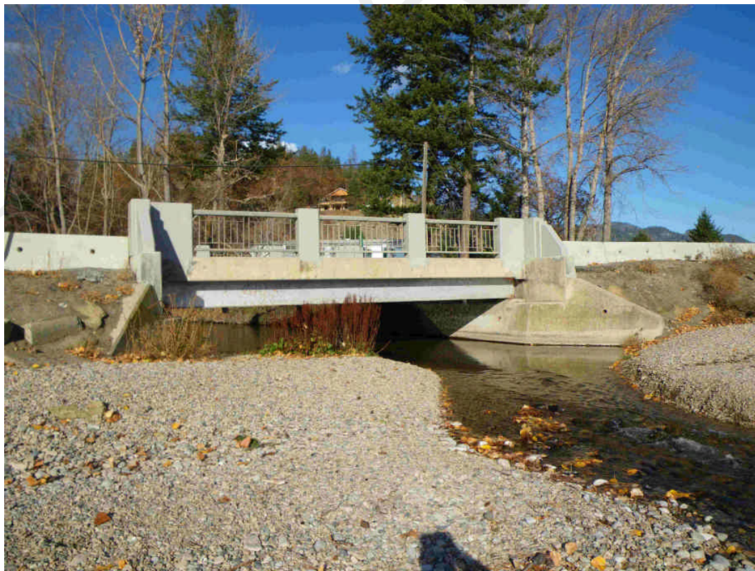
Photo 10. Highway 97 Bridge over Peachland Creek on the fan. Note limited clearance.
