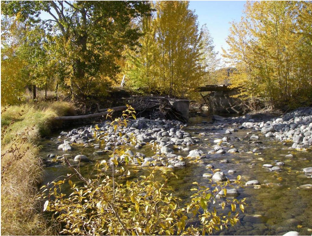
Photo 2. Abandoned public or private road crossing with approaches in active fan area downstream of CPR crossing. Washout likely during high flow periods with sediment input to fish bearing waters.
