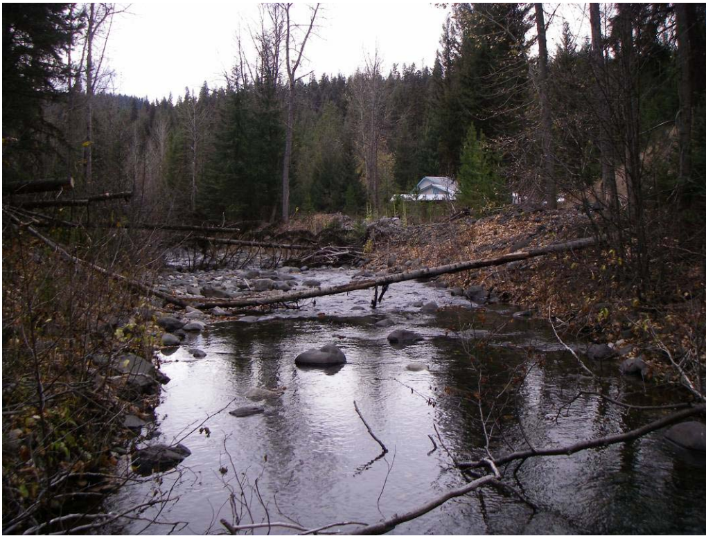
Photo 9. Private residence on fan upstream of upper Red Lake road crossing on Tranquille mainstem. Sediment and debris input to the canyon above results in accumulations on the fan during high flow periods with avulsion. The house was undermined in the spring of 1990.
