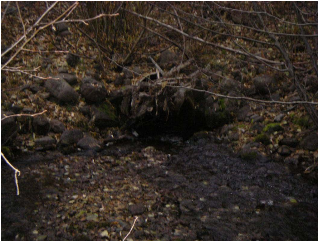
Photo 16. Mobile debris (log with rootball) at inlet of structure on Saul Creek at road K1100.35. Flows were overtopping the road in this location, resulting in diversion onto steep coupled slopes and erosion with input to Tranquille River.
