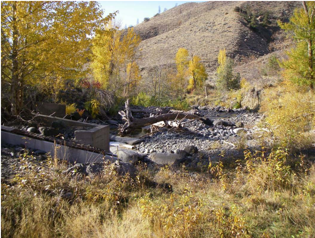
Old water intake infrastructure on lower Tranquille mainstem. The structure is a likely barrier to fish passage. Some water is still diverted from this site though existing infrastructure.
