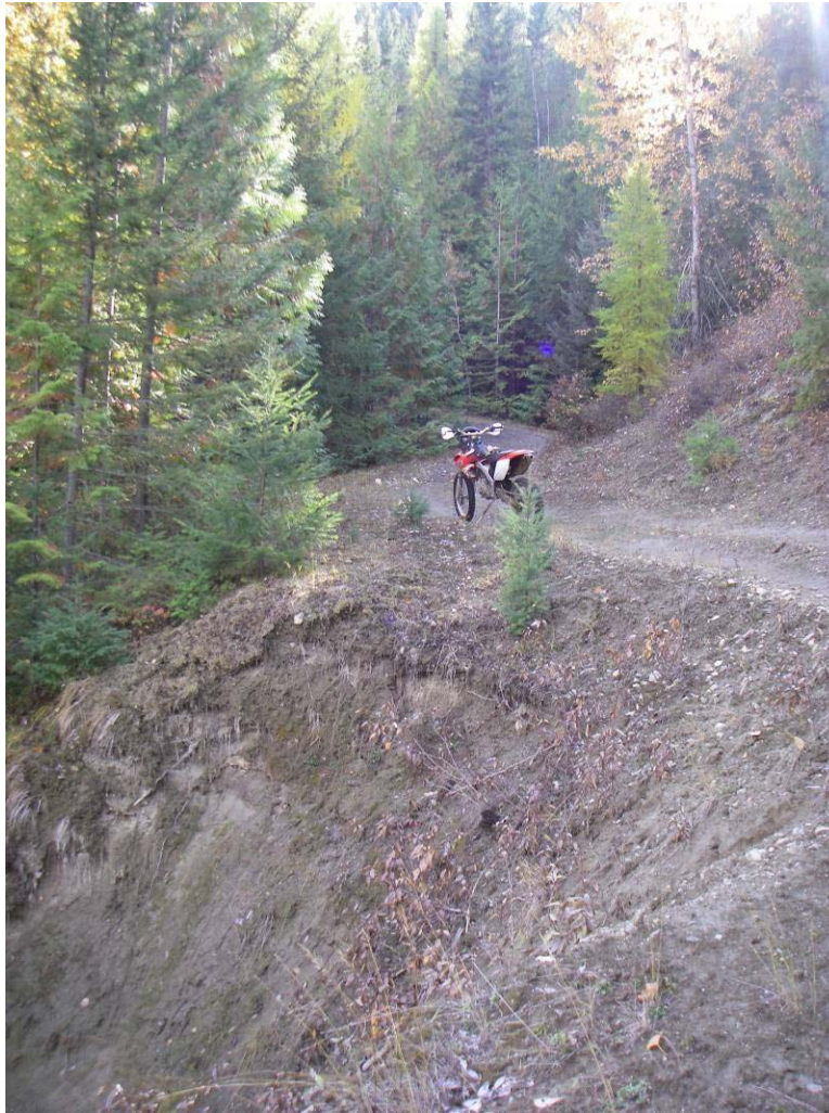
Photo 3. One of several landslides into Harris Creek or tributaries from non-status roads built in or on glacio-fluvial and glacio-lacustrine terraces in the residual area. In this case South Harris non-status road. Drainage infrastructure is failing resulting in diversions into unconditioned areas connected to channels. In other areas oversteepened or supported fill is failing resulting in landslides into channels and onto the Harris Creek floodplain.
