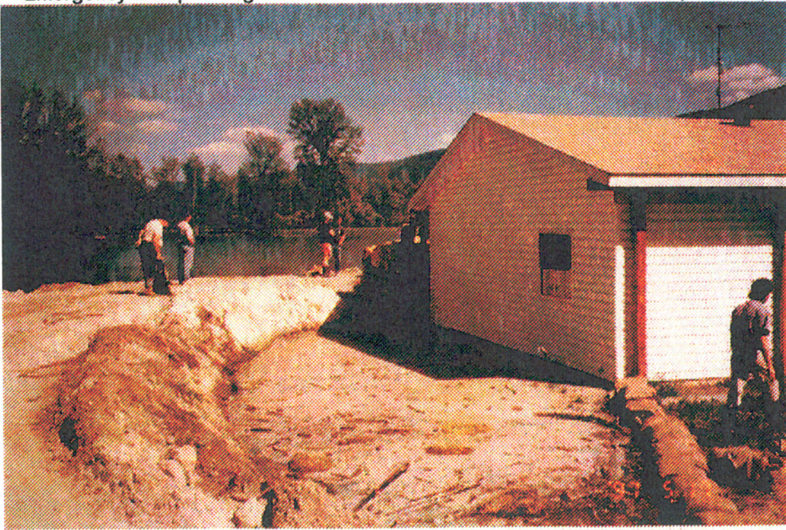
Emergency floodproofing-leftbank of Kettle River near Cross section 26 (HWM K6)
