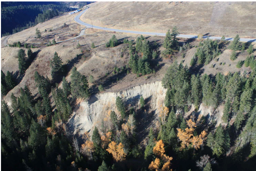
Photo 12. Typical large debris slump downslope of Highway 33 in lower Daves Creek.
