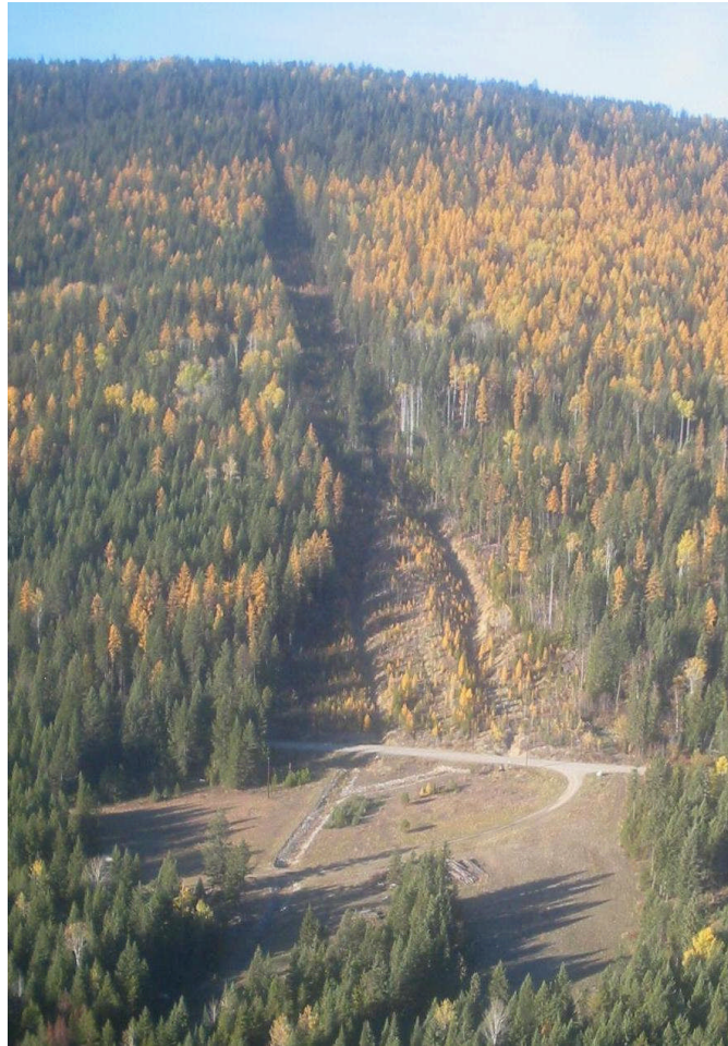
Photo 9. 1500m long, 17ha landslide responsible for 3 fatalities on Philpot Road in 1990, caused by drainage redirected along forest road.
