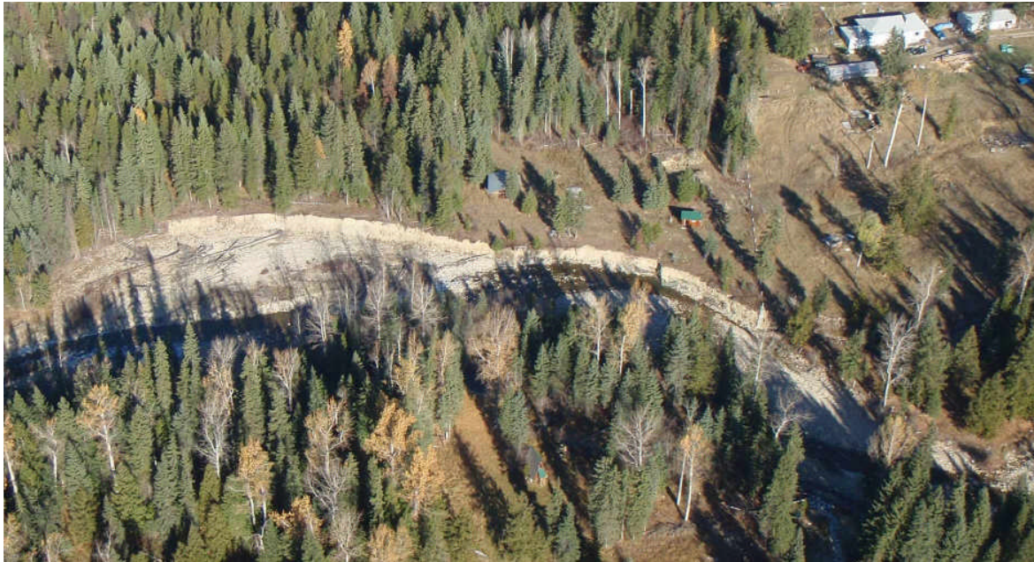
Photo 7. Mission Creek (Reach 5) bank erosion of thick sand, gravel and cobble glaciofluvial and fluvial sediments.
