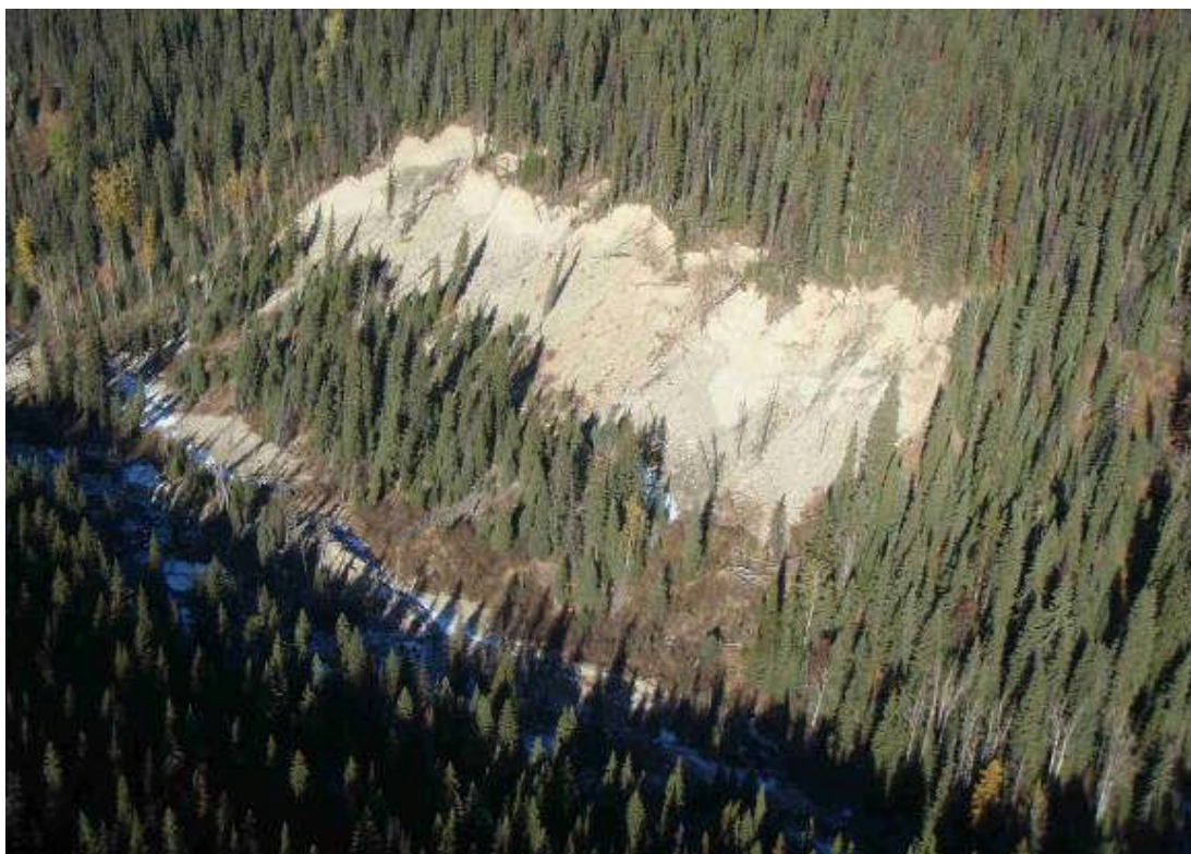
Photo 4. 250m long debris slump in Reach 6 Mission Creek. Initiated during 1997 high peak flows.
