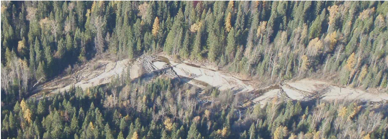
Photo 13. Reach 6 Mission Creek, aggraded and widened (Oct 27 2008)
