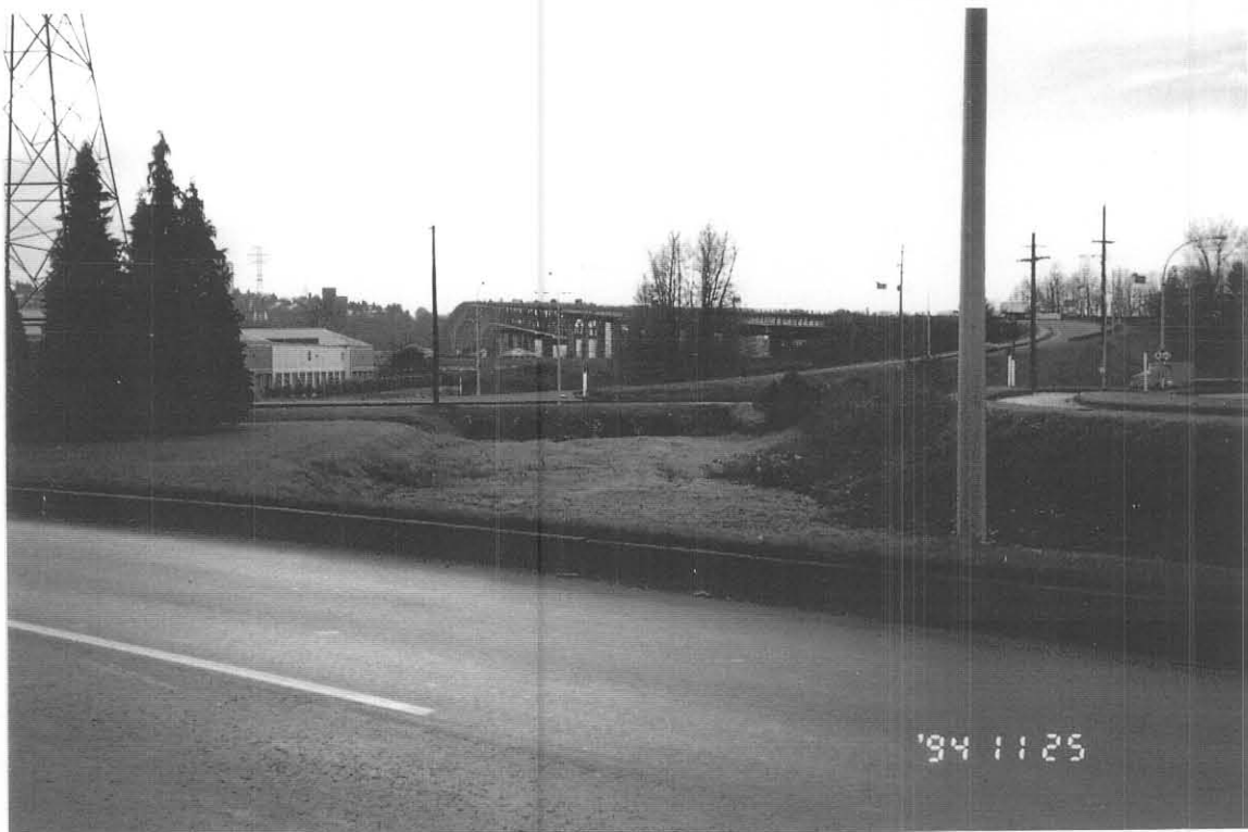
4. Looking downstream (south) on the drainage channel from Seymour Creek Indian Reserve #2 at the downstream set of six culverts under the Dollarton Highway and Highway 1 offramp.
