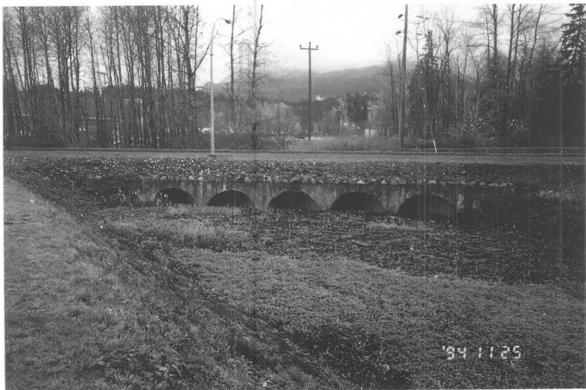
5. View upstream on the drainage channel from Seymour Creek IR #2 showing upper six culverts under the Dollarton Highway offramp to Highway 1. Seymour Creek IR #2 beyond roadway.
