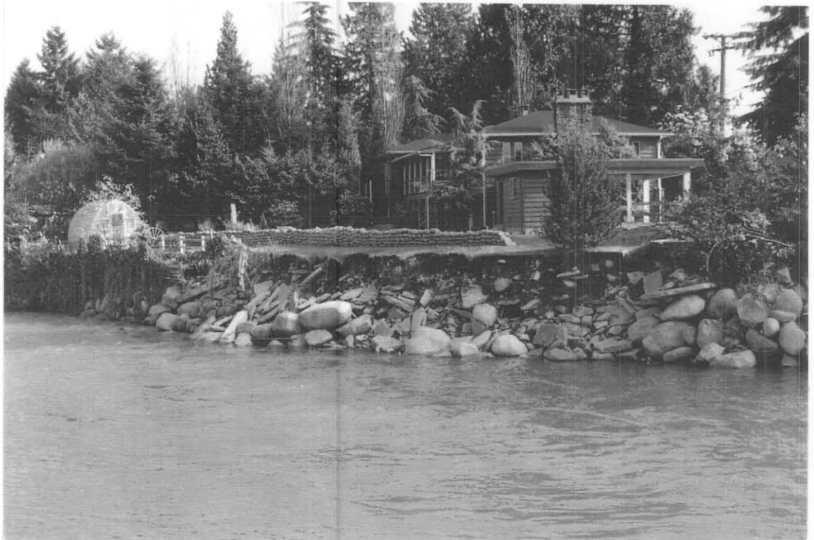
10. Looking upstream to the left (east) bank at XS-8 upstream of the Dollarton Highway bridge following the October 31, 1981 flood of record. Note severe bank erosion and sandbags on lawn.
