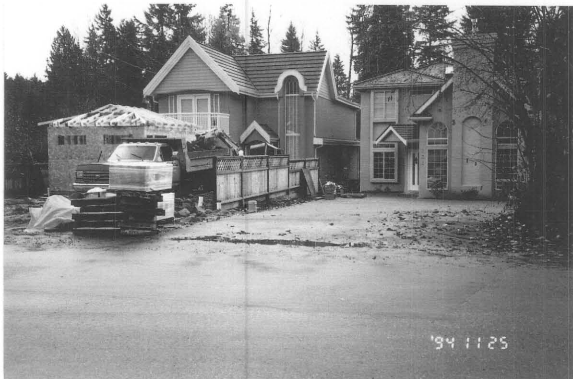
18. Looking southeast at 734 Seymour Boulevard and its' upstream neighbour. These homes appear to be constructed above the natural ground elevation.
