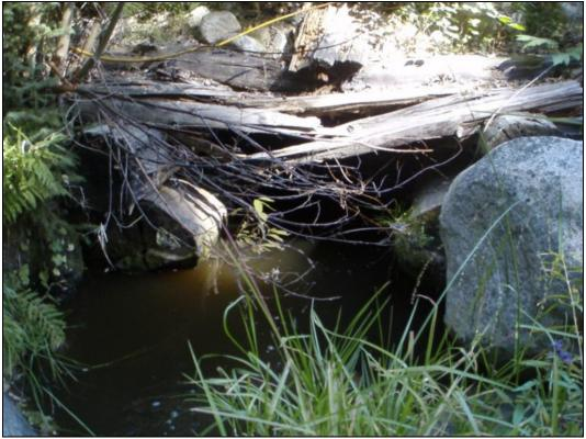
Photo 10 – Failing log culvert at Site 81 on mainstem of Paynter Creek
