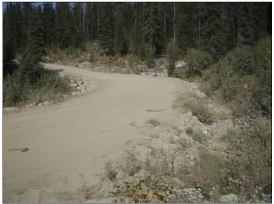
Photo 20 – Fine textured soils at Site 37 on active haul road near Bit Creek
