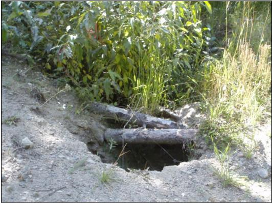
Photo 17 – Failing wood culvert at Site 51
