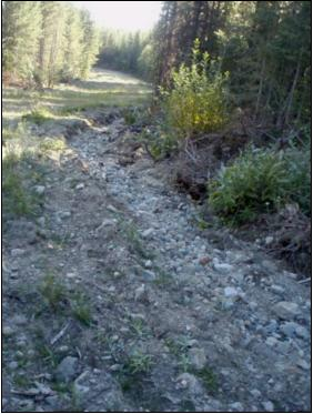
Photo 19 – Ditch erosion at Site 72
