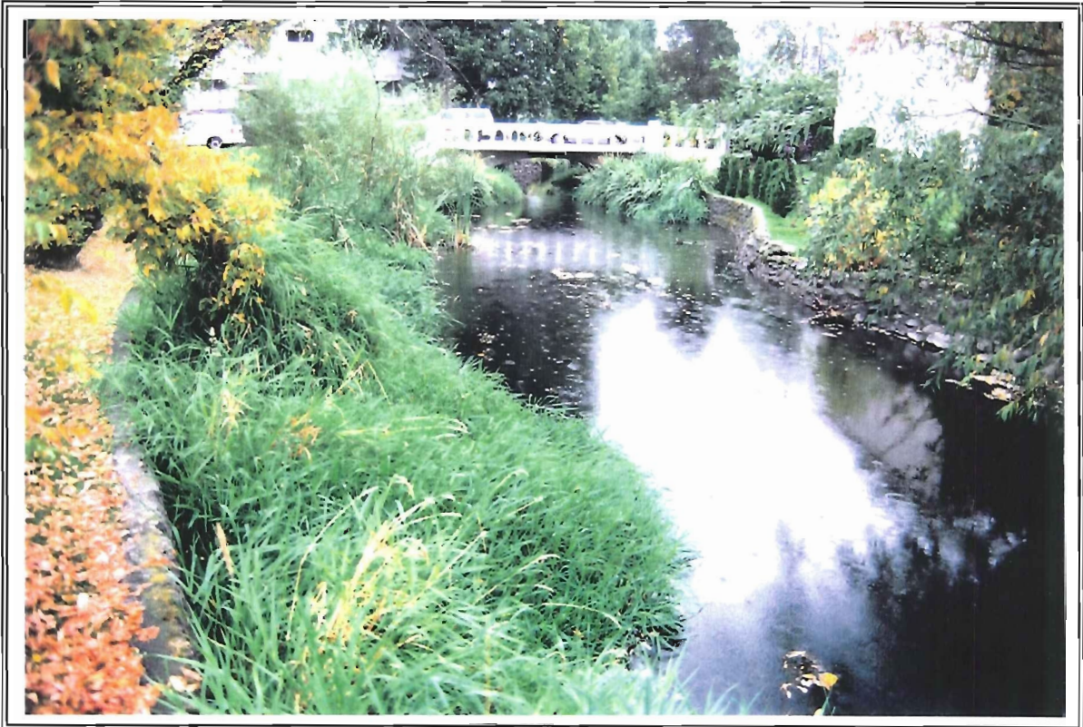
Upper section of Kelowna Creek within the study area. Note the retaining walls along both banks of the stream.
