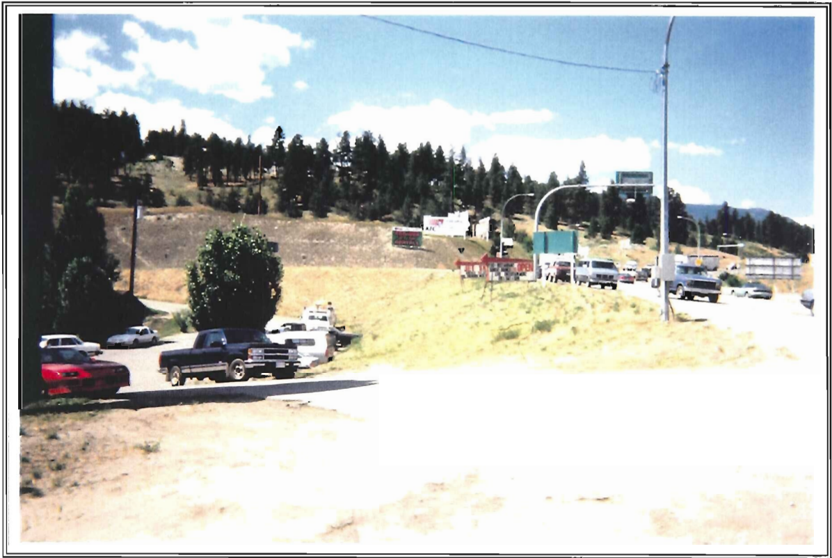
Upslope areas have been cleared for road and parking development.
