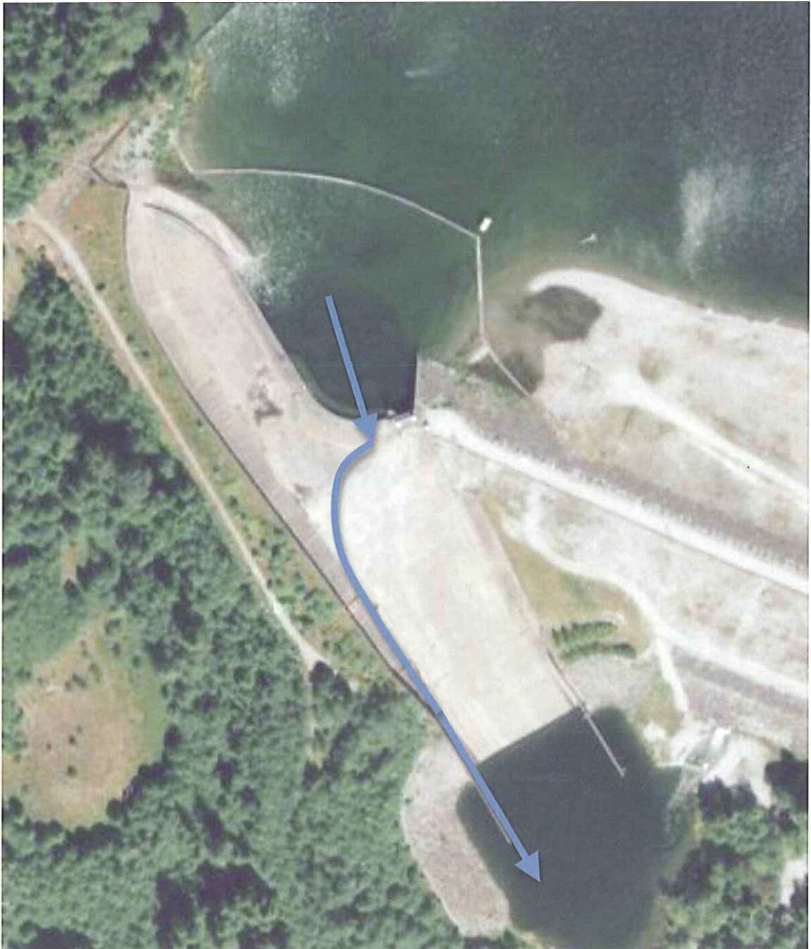
Figure 6. Google Earth satellite plan view of Alouette Dam, (Option 1 routing), showing locations of upper ladder (top arrow), connecting (curved) channel on spillway, and lower ladder (bottom arrow). Upstream fish movement will be against the direction of the arrows.
