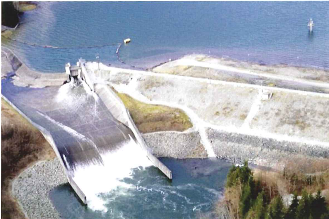
Figure 3. Alouette Spillway with a substantial discharge from the crest gate
