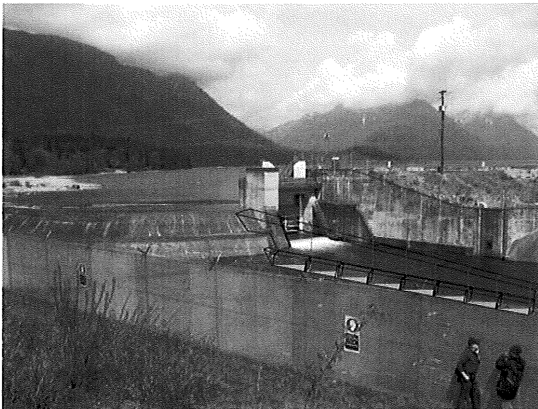
Figure 13. Eastside Spillway example showing ladder catering for variable lake levels
