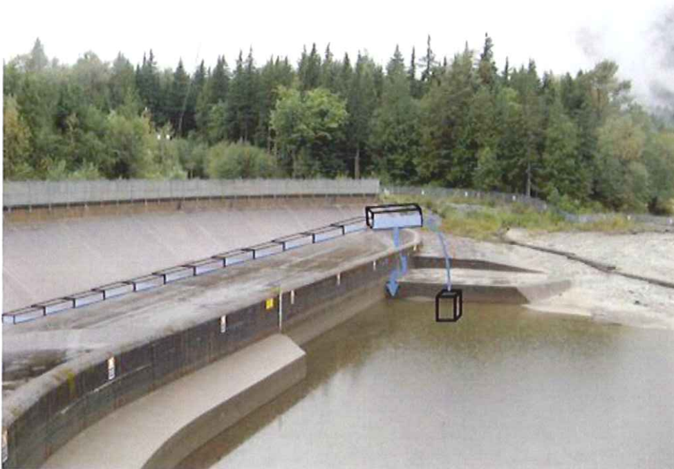
Figure 10. Westside Spillway example, showing pumped flow to small reservoir, and fisheries return flow to lake. Ladder will pass down west side of spillway.
