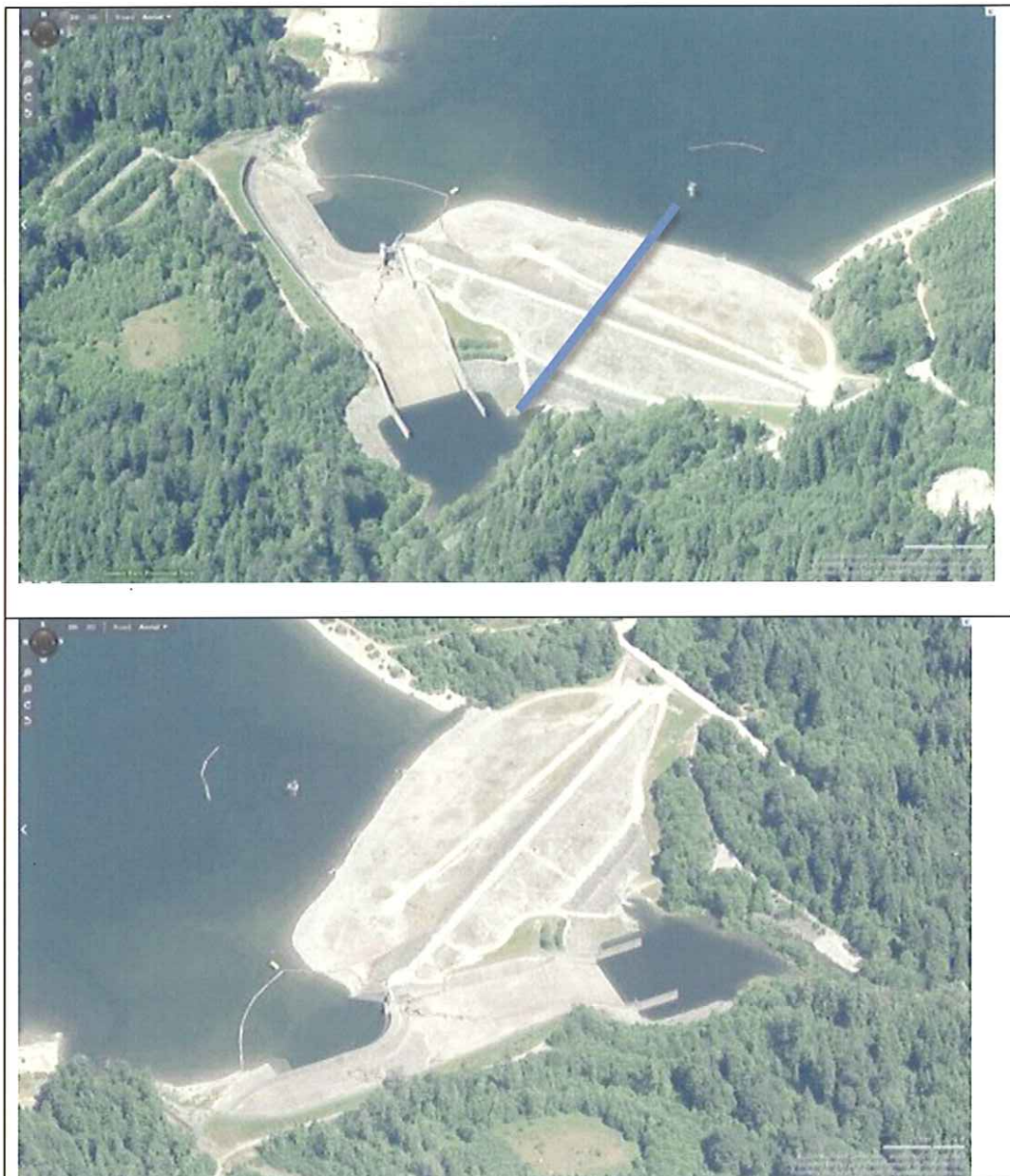
Figure 2. Bing Satellite Views: Alouette Dam and Spillway, looking north (top), and looking east (bottom). Lower Level Outlet pipeline route for fisheries flows shown (blue line).
