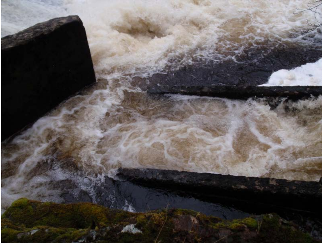
Picture 2. Entrance to Kloiya River fishway.
