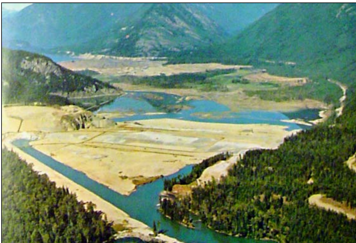
Figure 41: Construction of the Duncan Dam (photo BC Hydro library).
