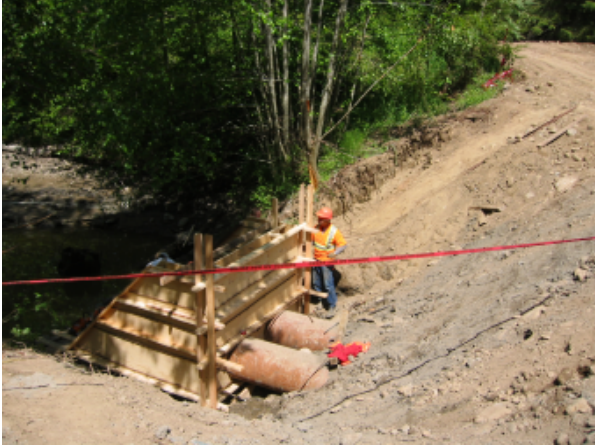
Figure 2 – Trash Rack Formed
