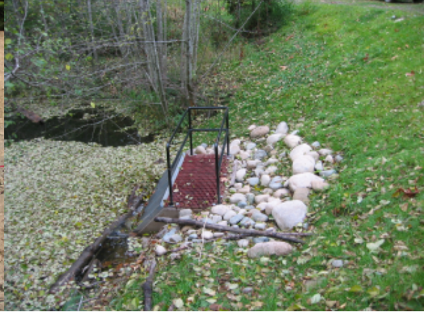
Figure 3 Trash Rack Complete
