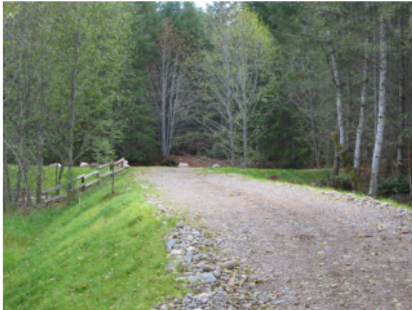
Figure 6 Completed Dyke – Settling Pond
