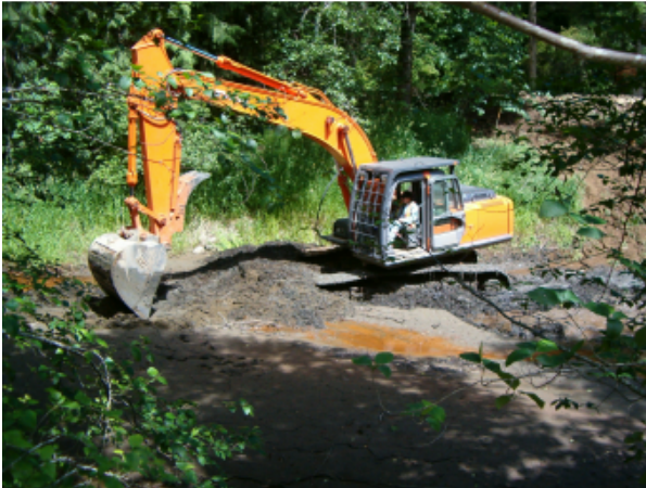
Figure 12 Dredging the Settling Pond
