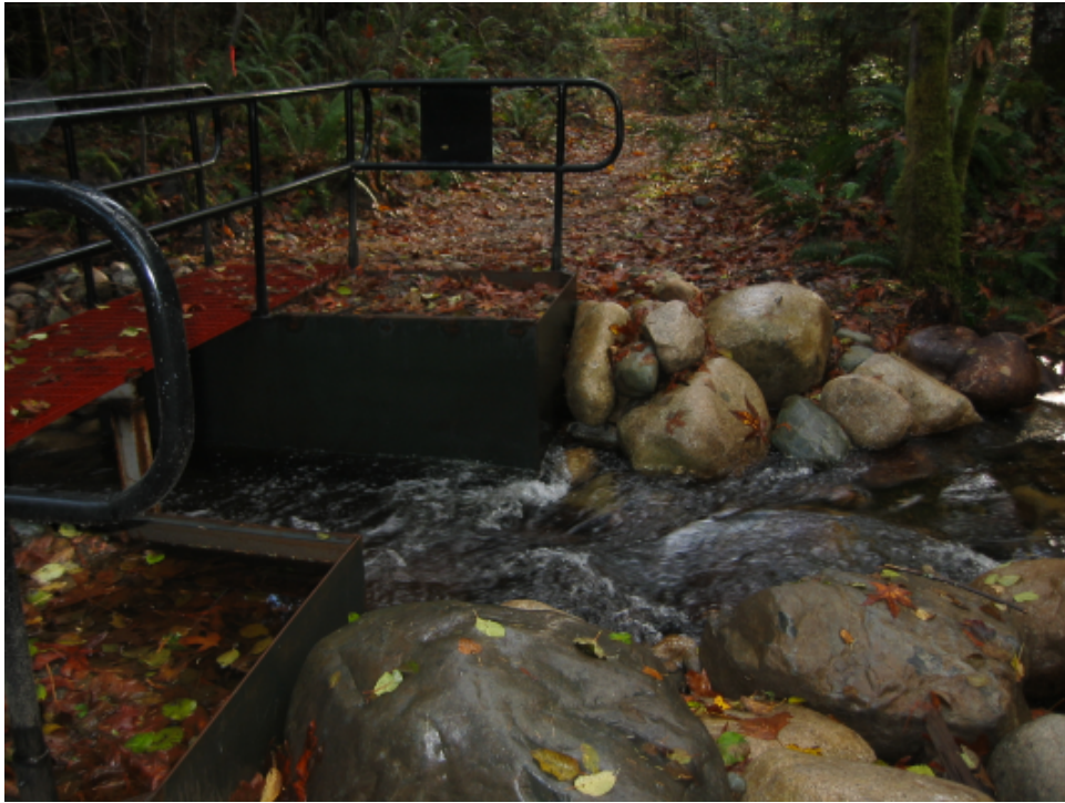
Figure 17 Downstream Fence Sill
