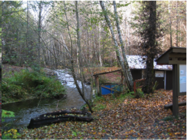
Figure 15 Newbury Weir Downstream
