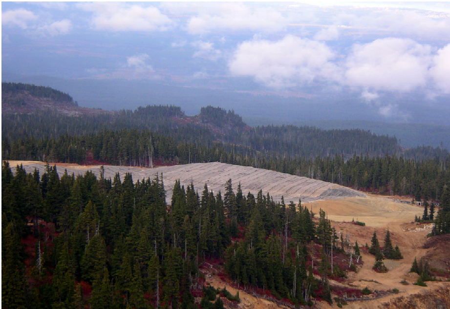
Figure 17. Geotextile membrane covers the Mt. Washington mine site September 2009. K. Campbell photo
