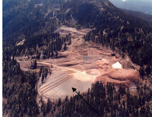
1999 – shows the partial cap installed in 1988/1989
