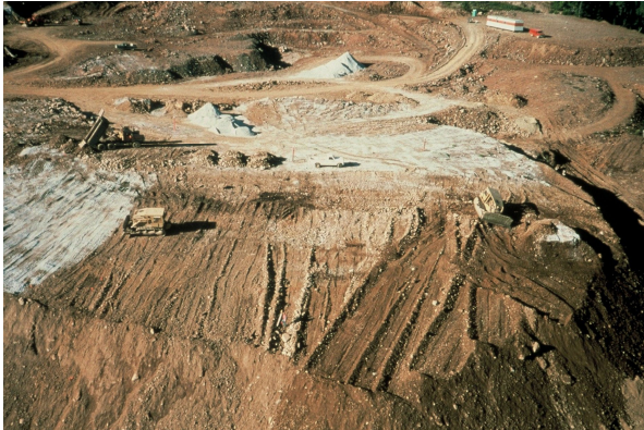
1988 – cleaning up the loose material and preparing to cover with gravel
