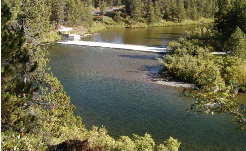
Figure 4. Steelhead enumeration fence and downstream holding pool. Photo courtesy of Brome and Leaf Steffey.
