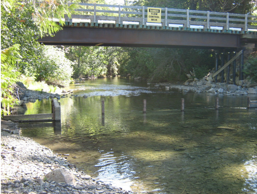
Photo 1. Pre-project conditions – note the fishway on the river's left.
