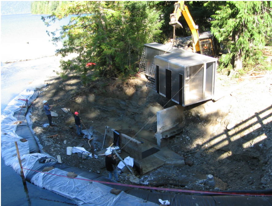
Photo 5. A hydraulic excavator positioned the fishway structure on the footings.
