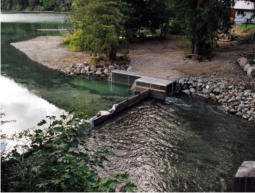
Photo 9. The gate was used to regulate flows in the river immediately after the construction was completed.
