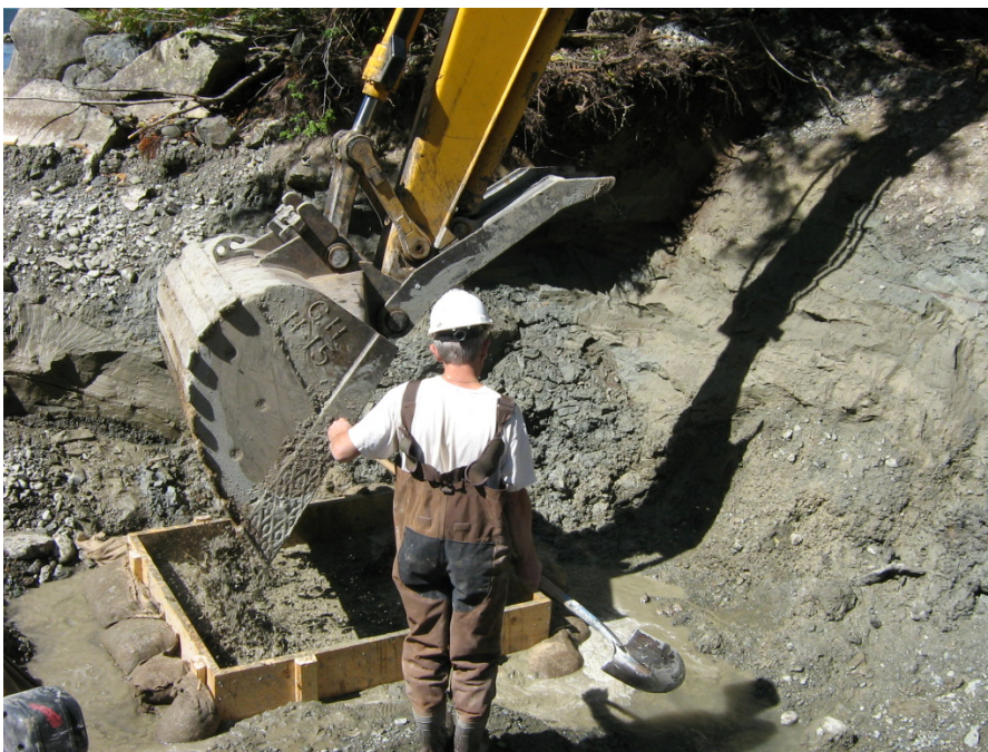
Photo 4. Reinforced concrete footings were constructed for the fishway structure.
