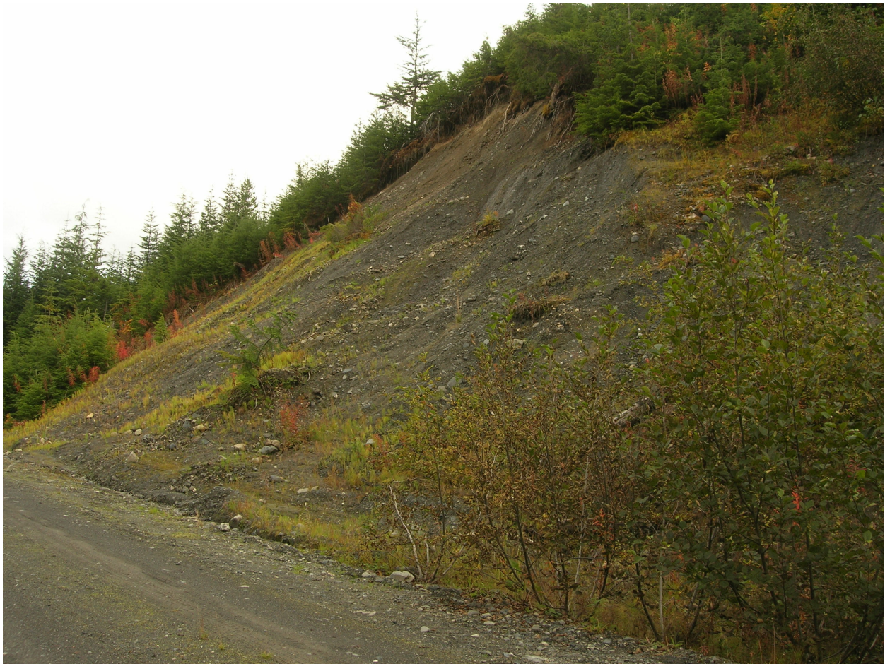
Photo 8: Site 186 - Looking at exposed RR cutbank needing revegetation. This was the largest of 4 areas of mass wasting near this crossing.
