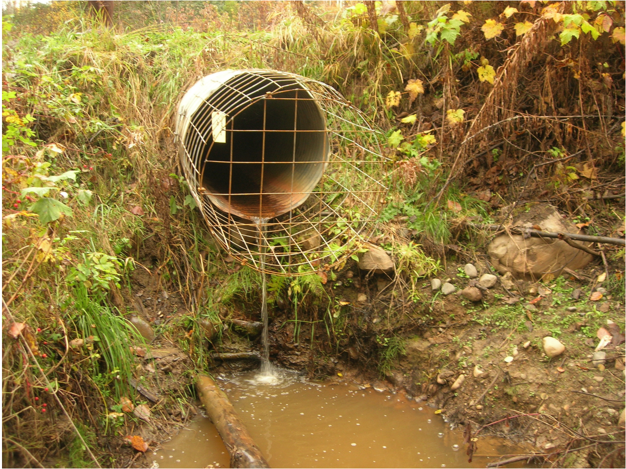
Photo 3: Site 270 - Looking upstream at culvert. Large culvert outfall drop evident, as well as beaver stop that would prevent adult fish passage. Turbid water from exposed banks visible.
