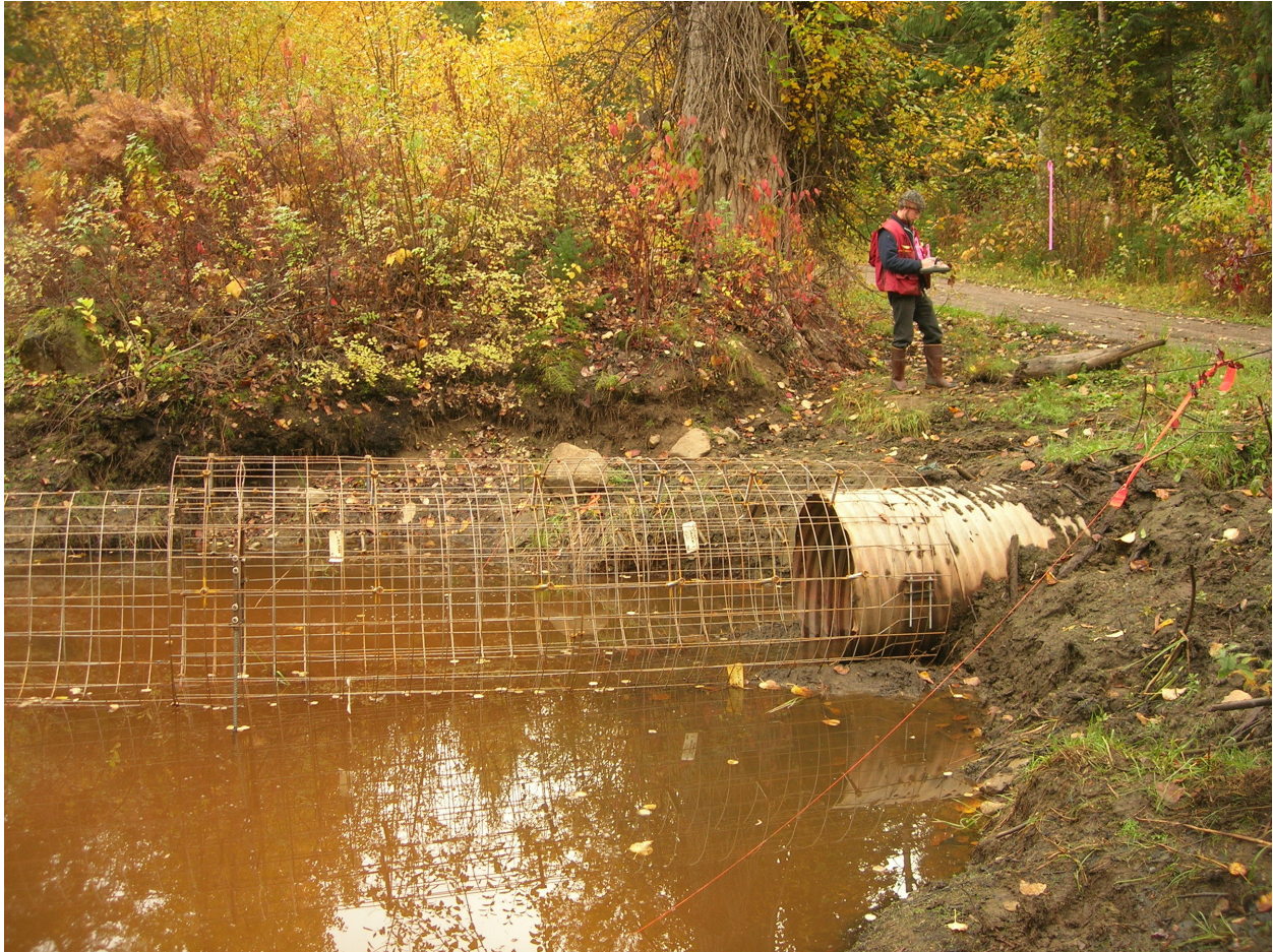
Photo 11: Site 270 - Looking across from right to left at culvert inlet. Silty water and exposed soil are evident.
