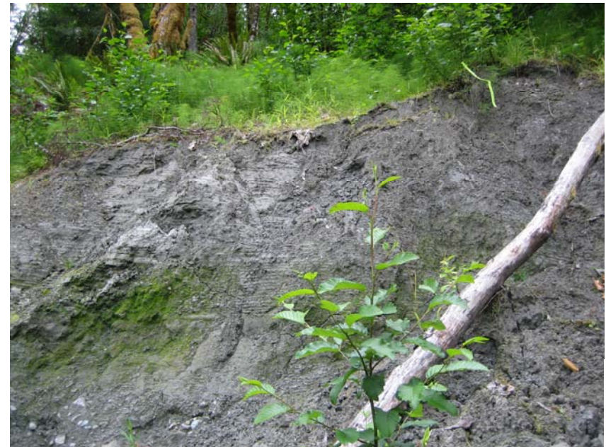
PHOTO 8 – OP #11 – Slide Scarp approximately 8m in Height July 7, 2009
