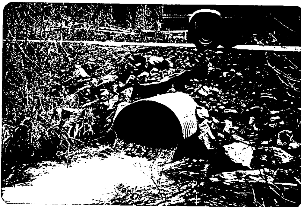
Cranberry River. Highway 37 culvert on McKnight Creek should be removed or replaced when new highway is built.
