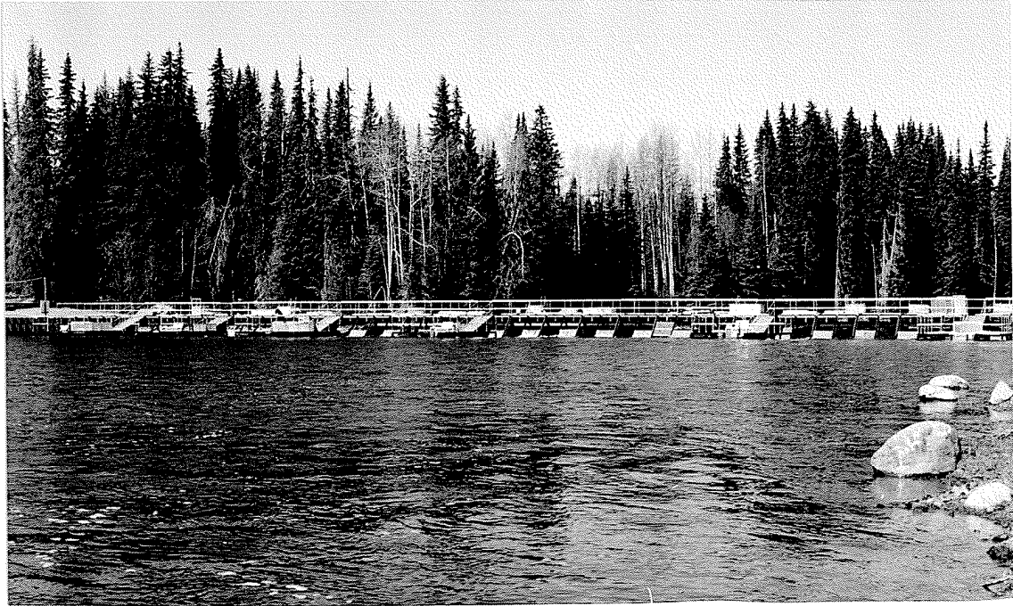
Figure 3. Photograph of the Babine River weir in May 1994. Note arrangement of fence panels.
