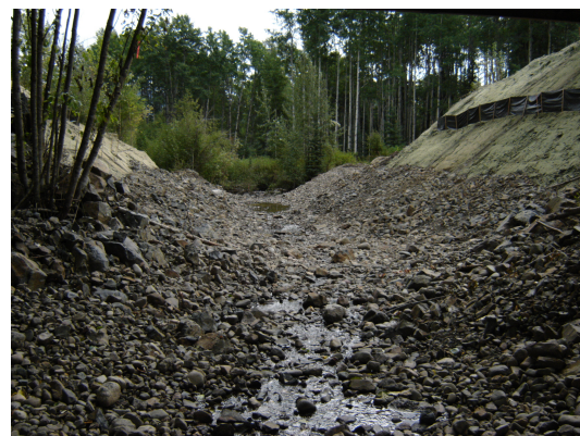
Photo 3. View of New Channel Looking Downstream.
