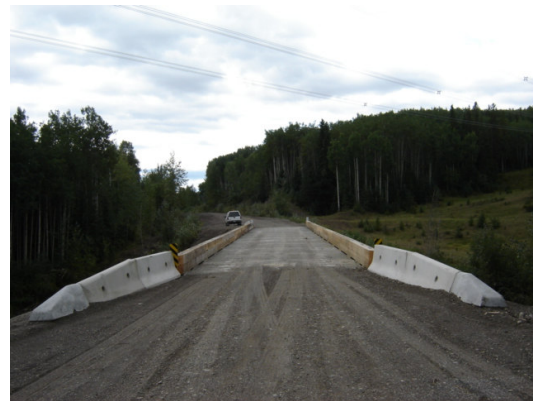
Photo 2. New Barren Creek Bridge
