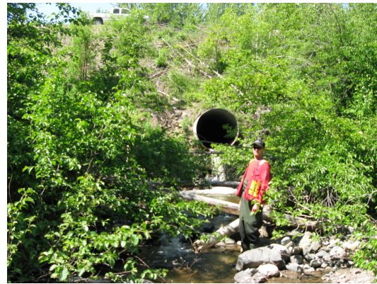
Photo 1. Stream Culvert Outlet.
