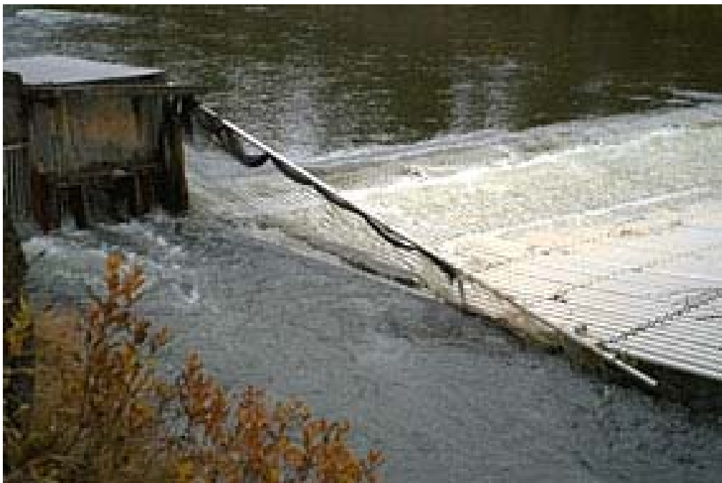
Photo Figure 8. View from right banking of aluminum pole holding up panel netting.
