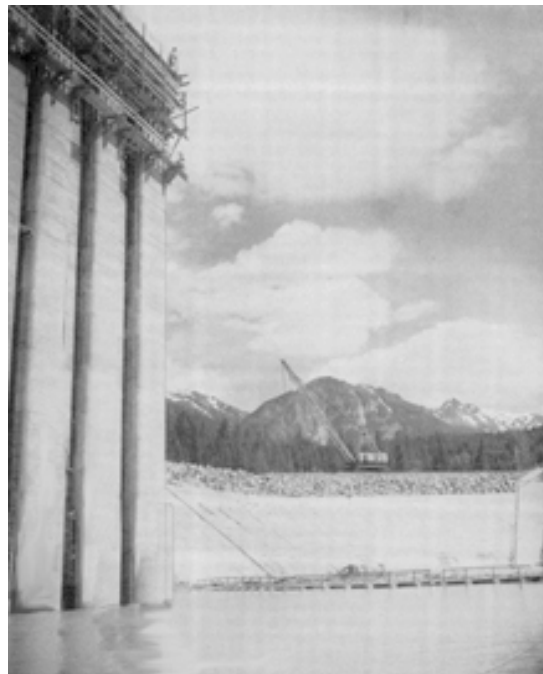
Figure 10-3. La Joie Dam under construction (Water Powers B.C. 1954)
