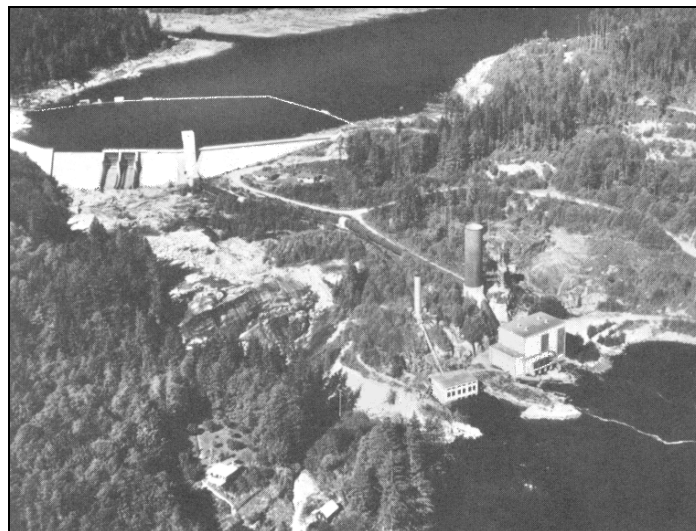
Figure 14-2. Clowhom Dam (BC Hydro)
