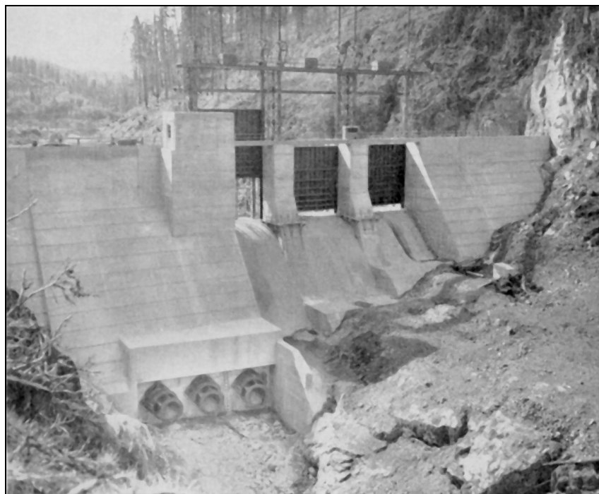
Figure 2-4. Ladore Falls Dam (BC Power Commission)
