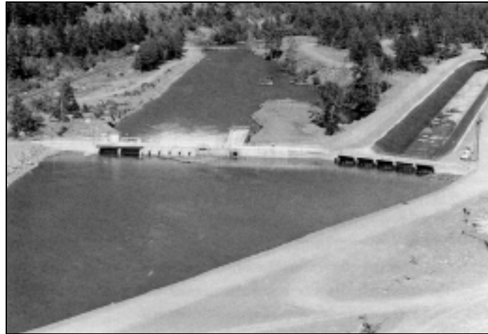
Figure 11-1. Seton Dam nearing completion about 1955 (Roos 1991)
