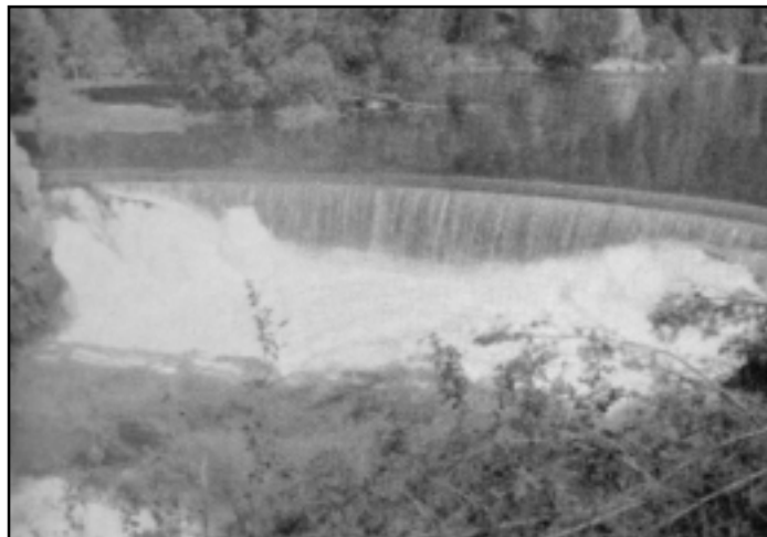
Figure 12-3. Wilsey Dam (Water Powers B.C. 1954)
