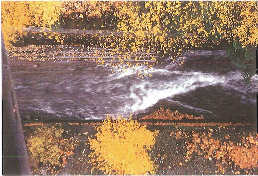
Figure 6. Upper portion of flume under the railway crossing at the top of Kwoiek Creek Reach 1 (viewed from above).
