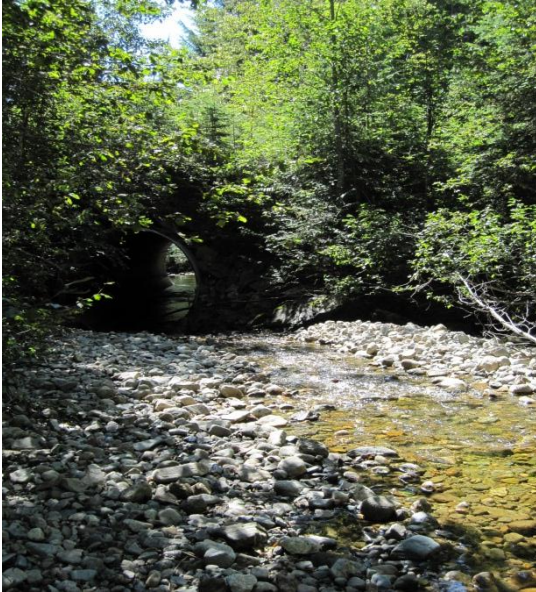
Photo 5. Stevens Creek above FSR culvert
