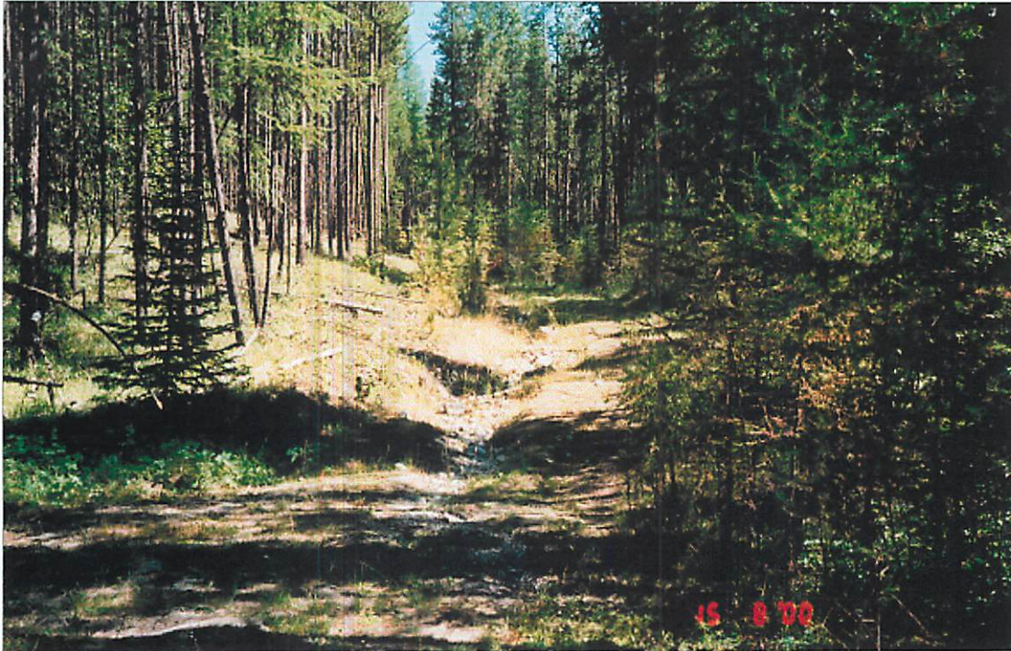
Photo 21 - Old road in South Ellis Creek watershed not properly deactivated (field inspection site DWT99). Note meltwater channel in roadbed and lack of waterbars or culverts. Area was logged some time prior to the 1960s. Site is located roughly 70m upslope from failure shown in Photo 22.
