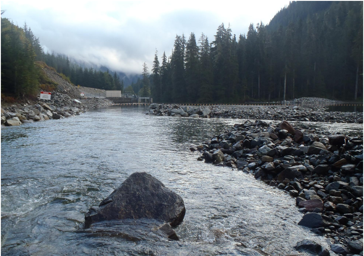
Figure 3.5 View of the Hydromax Energy UCRHPP intake and headpond.
