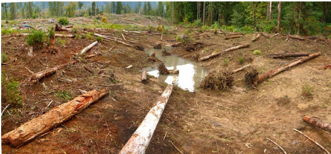
Partially filled wetland B post construction
