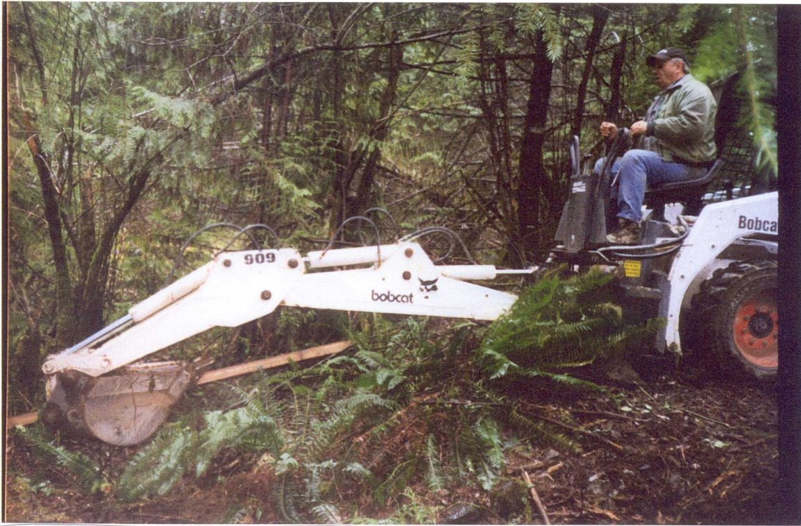
Figure 13. Small excavator installing posts for lead fencing, December 2002.
