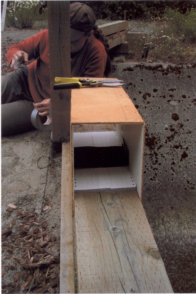
Figure 18. Track plates installed on overpass and bridge curb timbers (Fall 2004).
