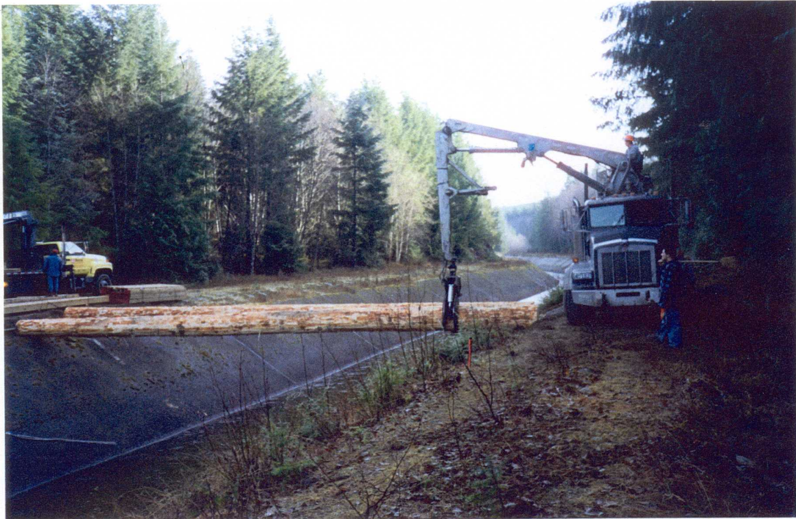
Figure 10. Mounting overpass stringers on mudsills, October 2002.
