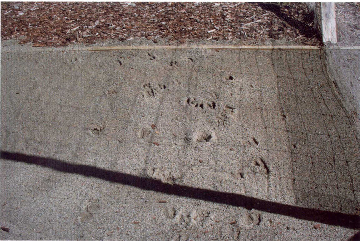
Figure 15. Track beds of sand installed on overpass approaches and mid-span.
