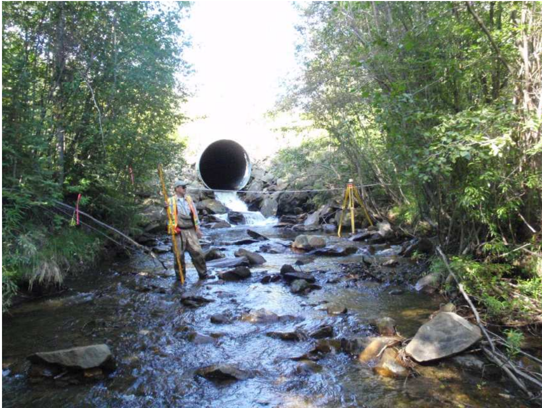
Photo 5. Looking upstream at cross section at chainage 0+069 m.
