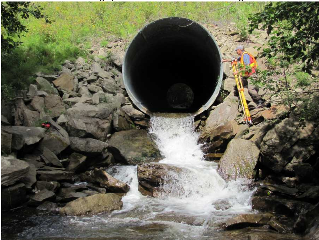
Photo 6. Looking upstream in Unnamed Creek culvert at chainage 0+086 m.
