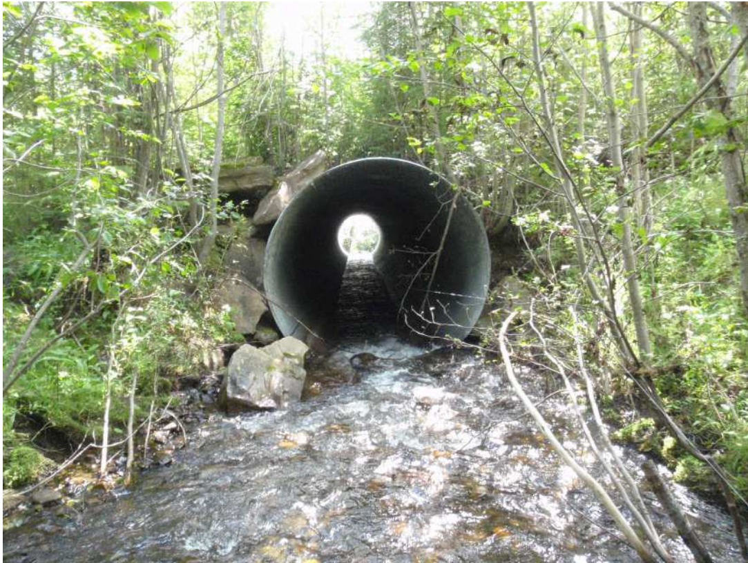
Photo 7. Looking downstream at culvert in Unnamed Creek from chainage 0+130 m.
