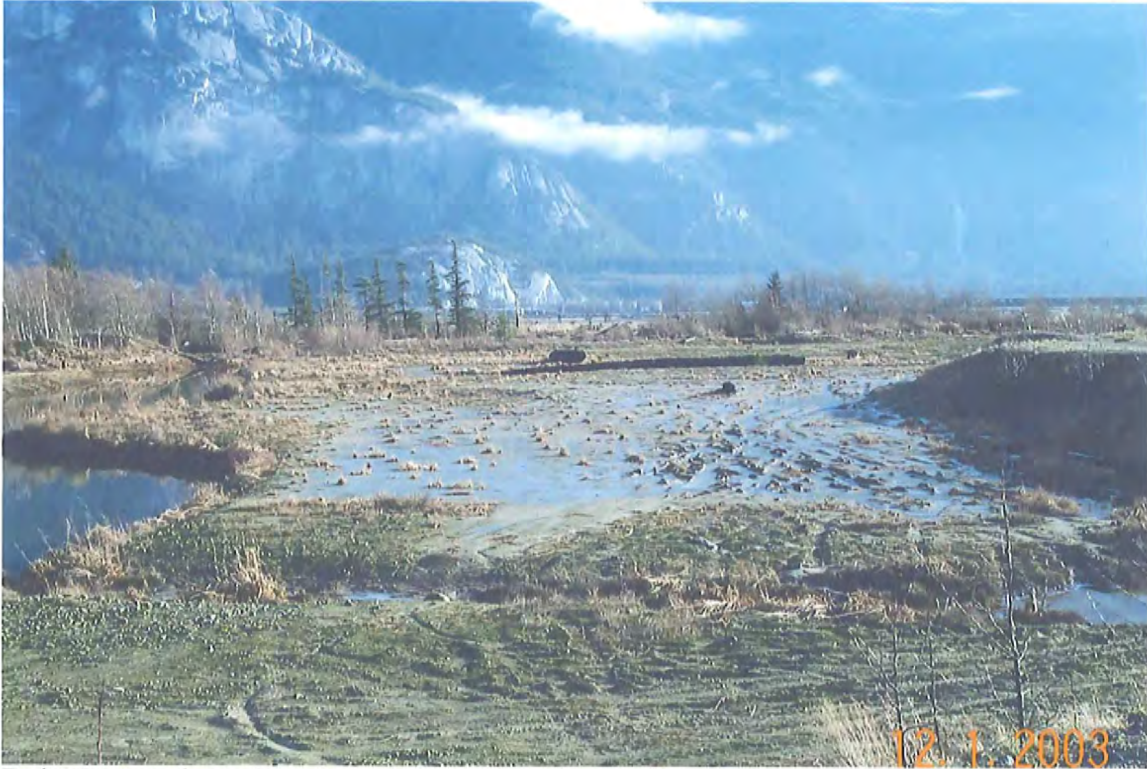
Facing East – sedge replant on graded estuary flats (berm/trail on right)
