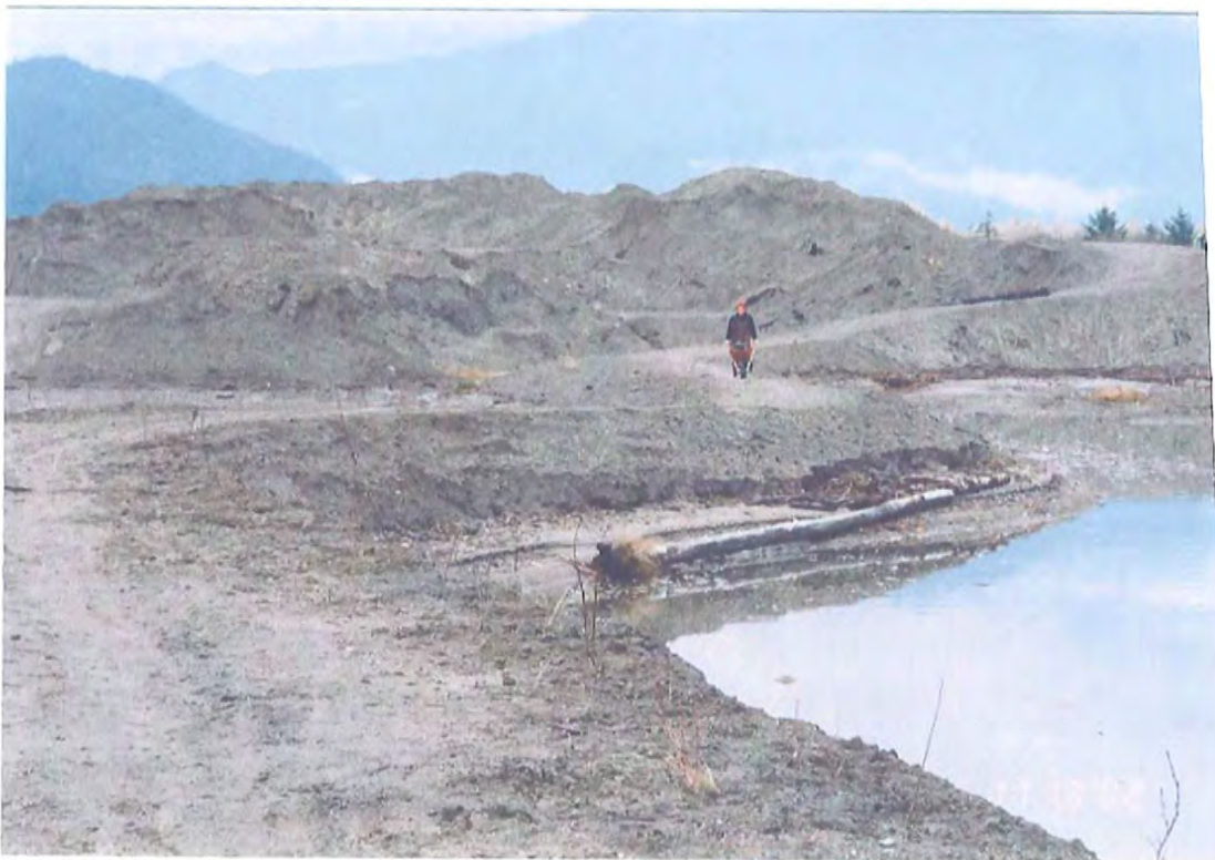
Facing North - a closer view of the dredge spoils with crew member
