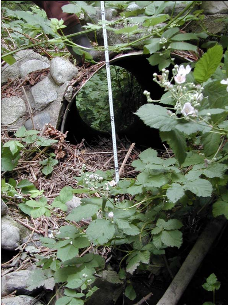
Figure 26. Upstream view of culvert at site SI 175 on Latimer Creek.
