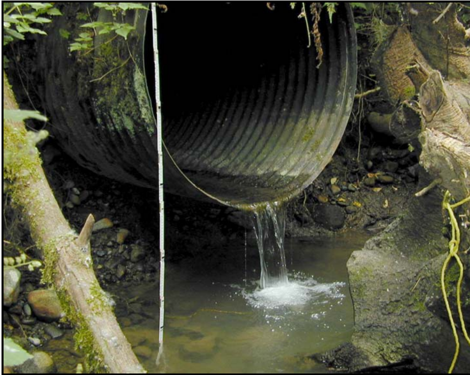
Figure 30. Downstream end of culvert at site CU 382 on Latimer Creek.
