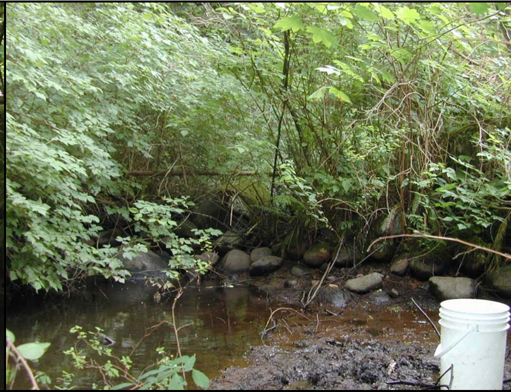
Figure 21. Dam and culvert at site SI 170 on Dogwood Creek.
